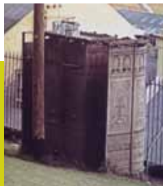
Cast iron urinal on Observatory Hill in 1960 before relocation to George Street (Photograph: City of Sydney Archives)
