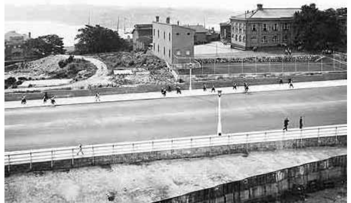
Fort Street Model School during construction of the Sydney Harbour Bridge, 1932 (Photograph: State Records)
