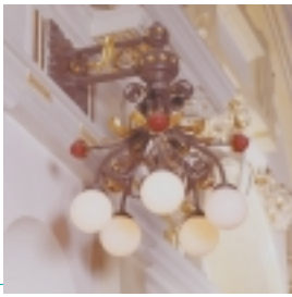
Wrought iron waratah pendant light fitting, Main Hall. Photo by Greg Piper
