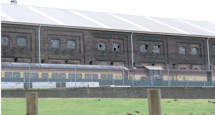
The Large Erecting Shop
