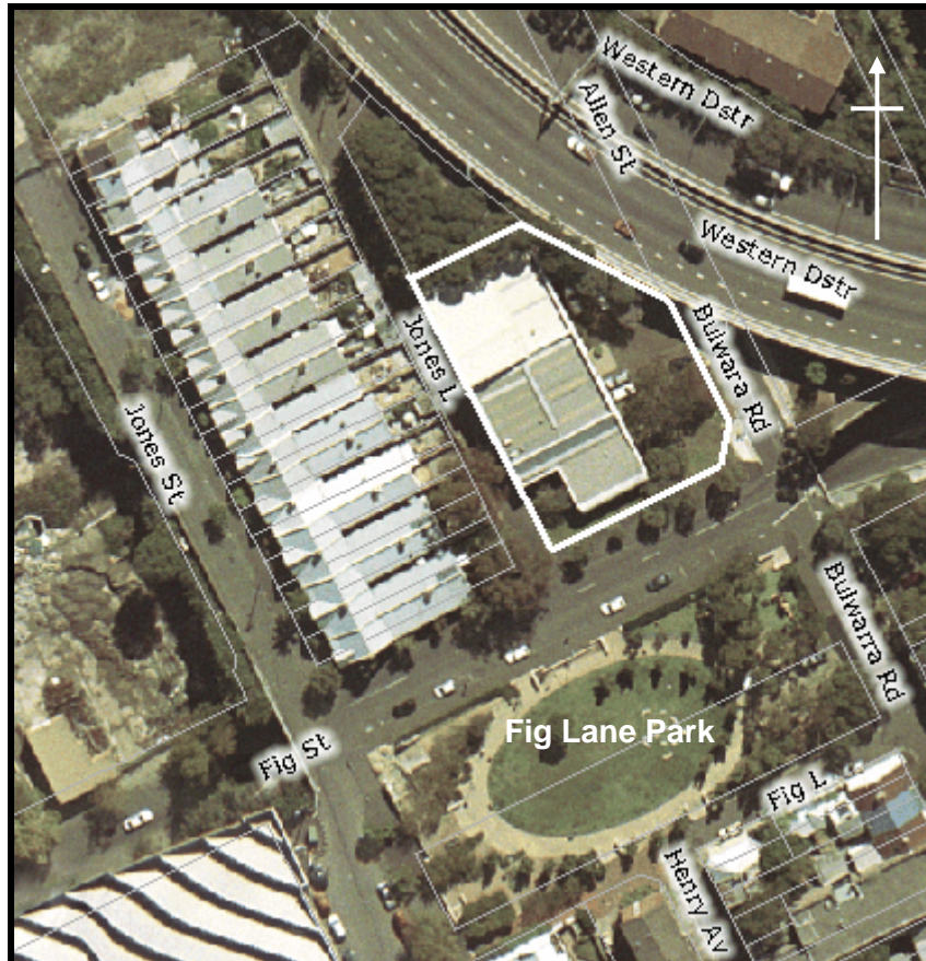
Aerial view of surrounding area, site perimeter is in bold with warehouse to be demolished shown.
