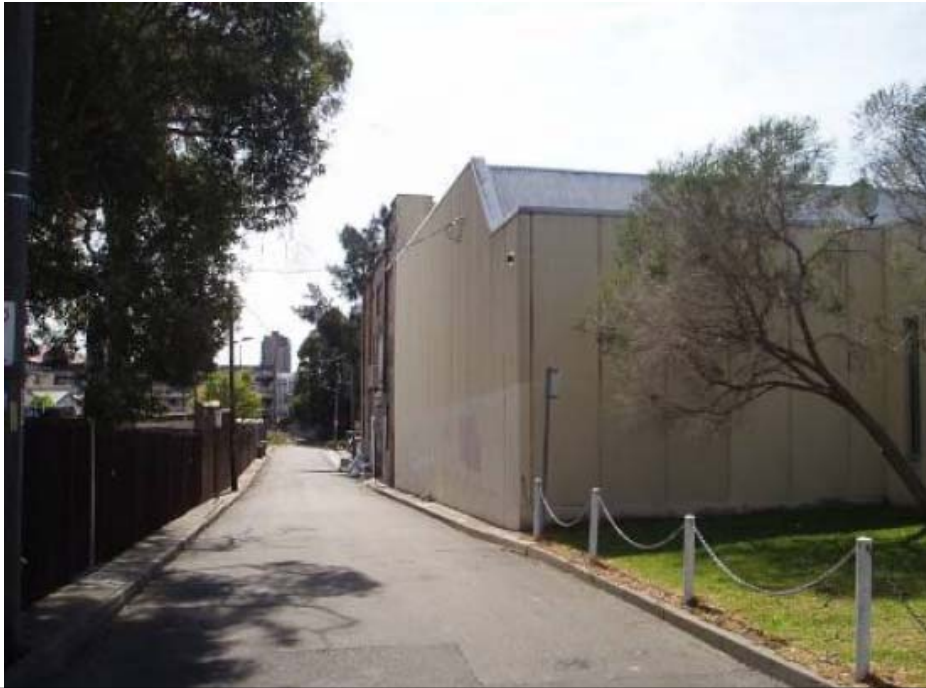
Looking north along Jones Lane. Building to be demolished is on the right with heritage terraces to the left.
