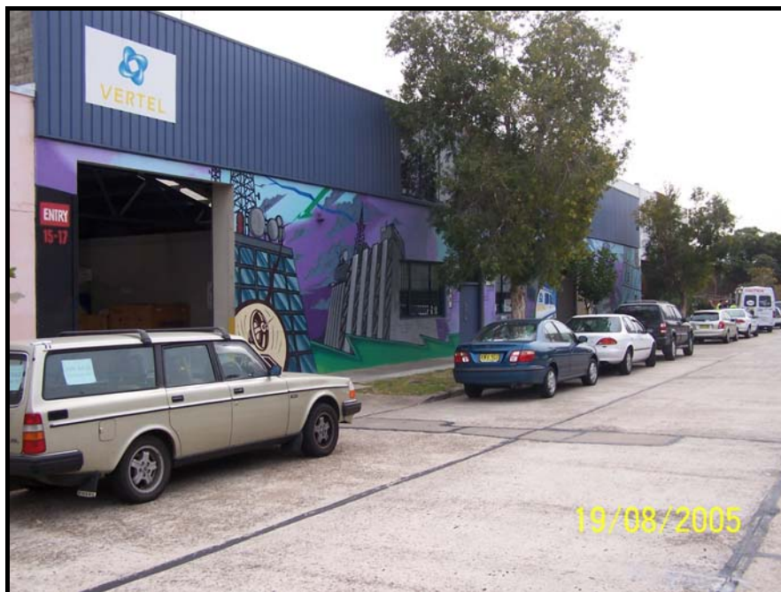
Photograph 3: Looking North along William St towards adjoining site (15-17 William St)
