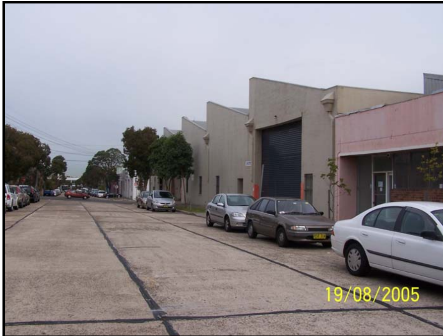
Photograph 2: Looking South West along William St towards adjoining site (21-27 William St)
