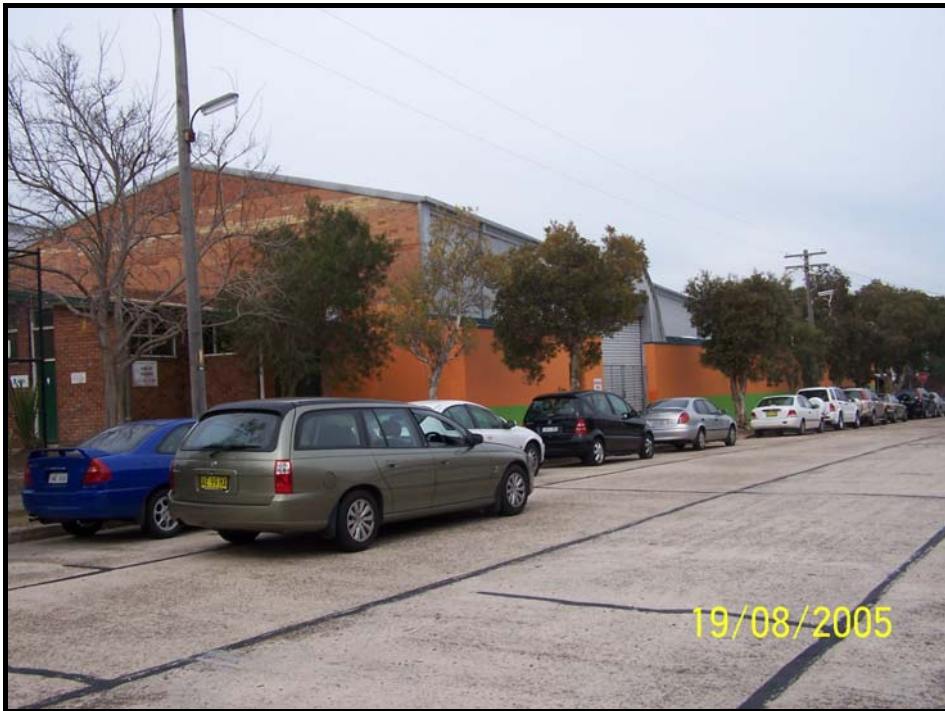
Photograph 4: Looking South-east along William Street towards Property known as 17-19 Collins Street, Beaconsfield
