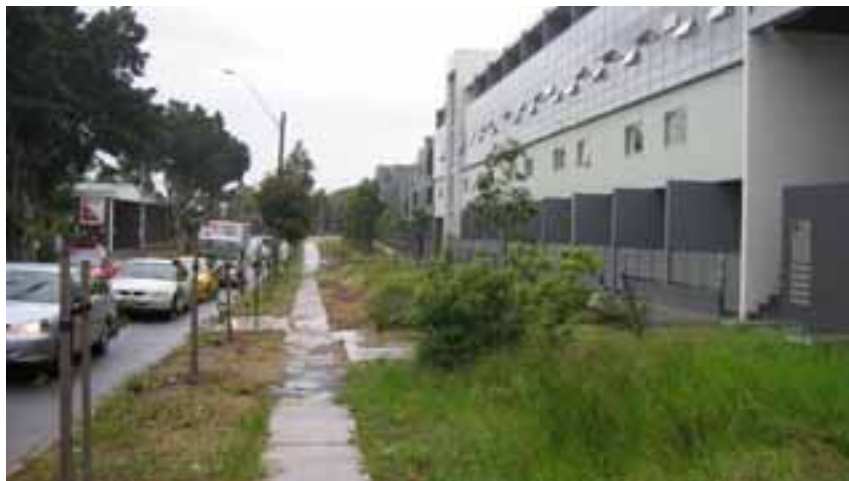
Example of soft landscape strip associated with new development on Euston Road which is a poor urban outcome.
