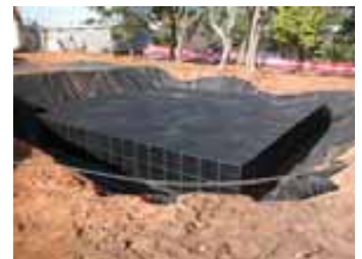
Example of detention tank system Source: Atlantis products.
