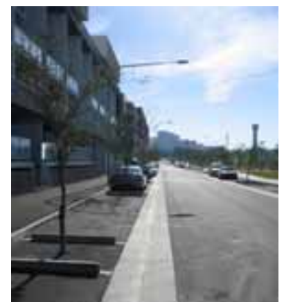
Example of residential with raised floor levels and negative relationships with the street.
