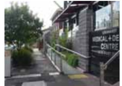
Example of raised entry off street.
