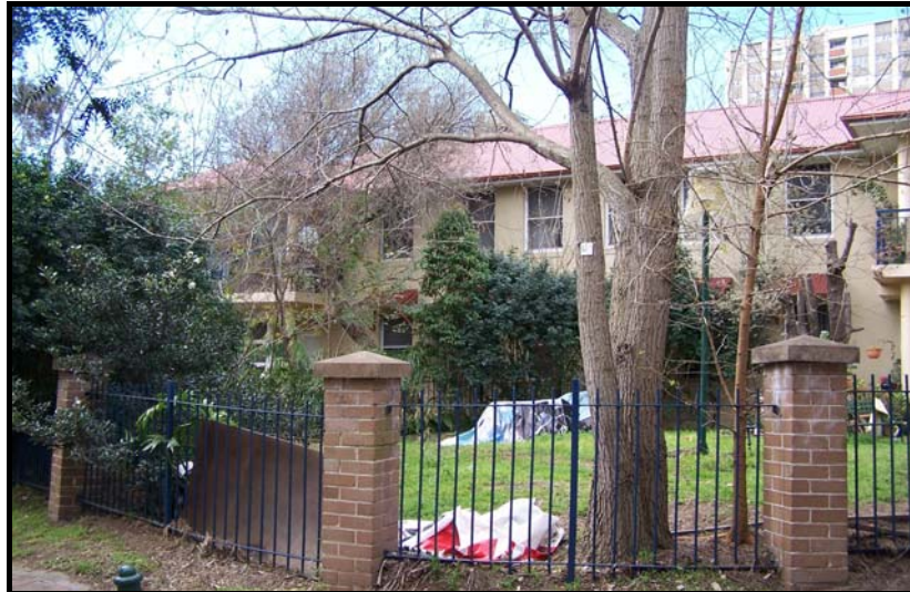
Figure 2: Subject site as viewed from the corner of Walker and Phillip Street
