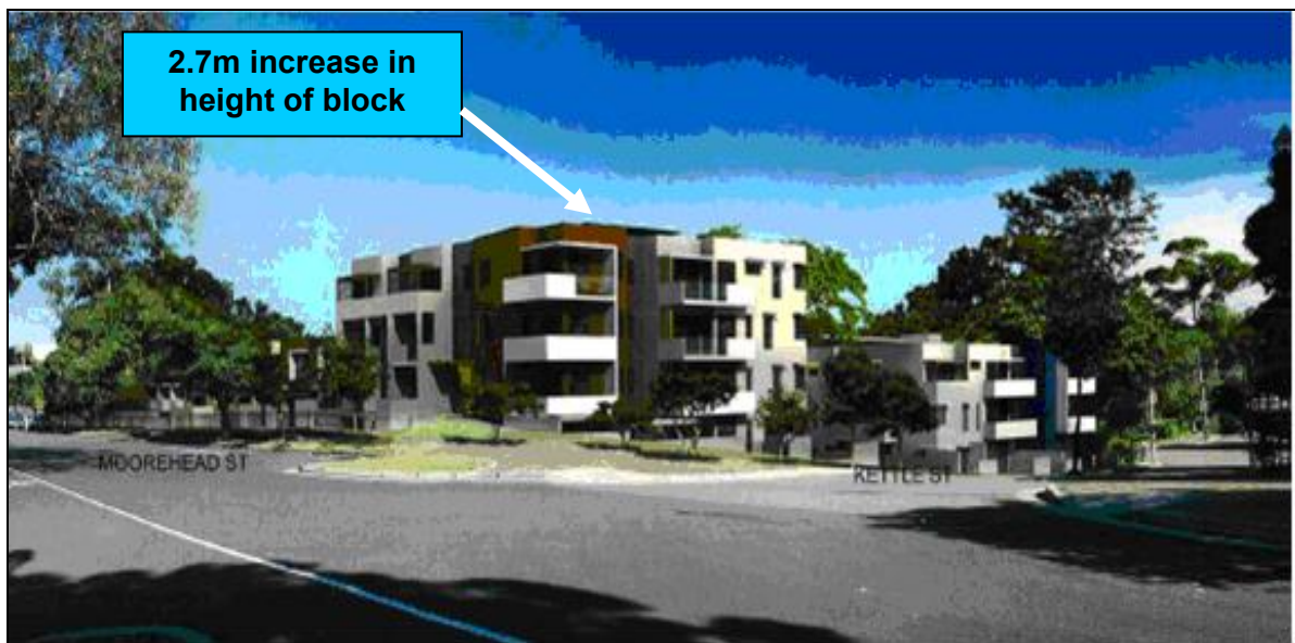
Figure 15: Subject site as viewed from corner of Morehead and Kettle Street.
