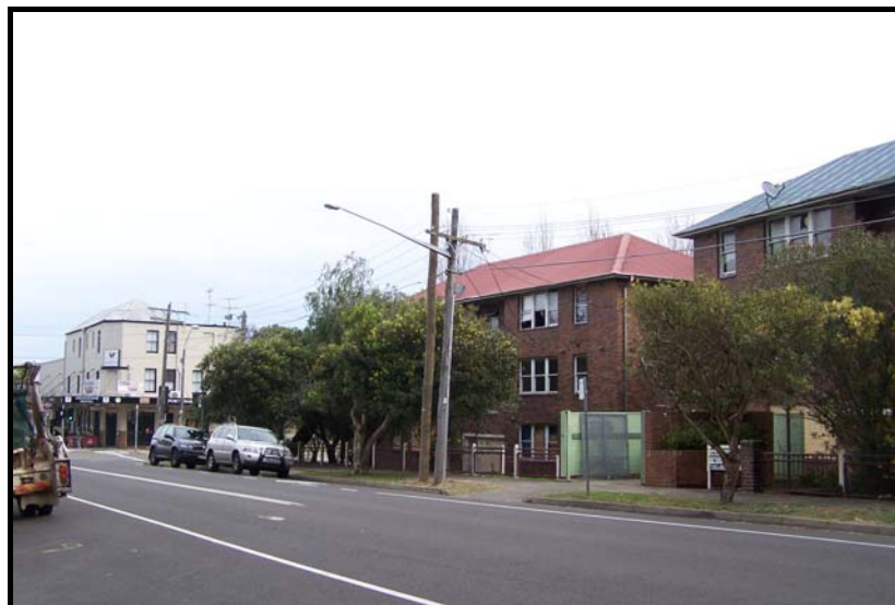
Figure 5: Opposite side of Morehead Street looking south.
