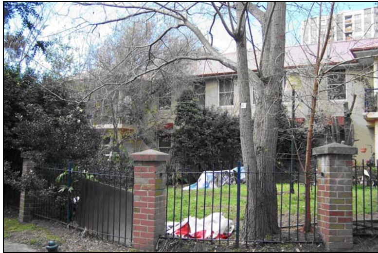
Figure 2: Subject site as viewed from the corner of Walker and Phillip Street
