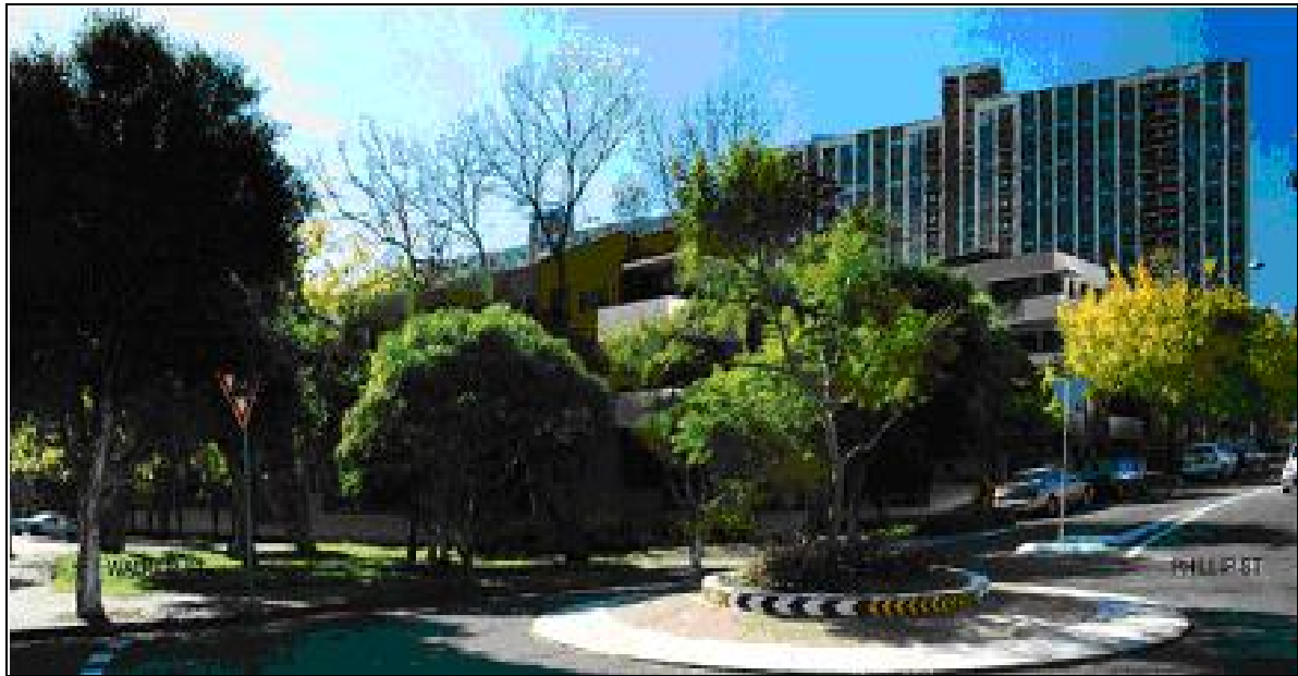
Figure 14: Subject site as viewed from the corner of Phillip and Walker Street
