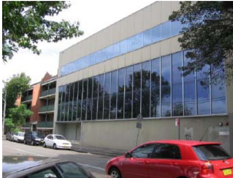
Figure 2 – Southern Street Façade of South Sydney Leagues Club with 4 Storey Red Brick Apartment Building adjacent to the Left
