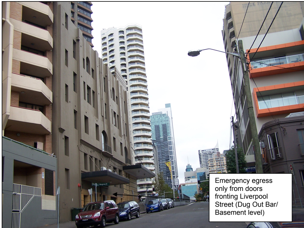
Photo 2: View of Burdekin Hotel from Liverpool Street showing emergency egress point.
