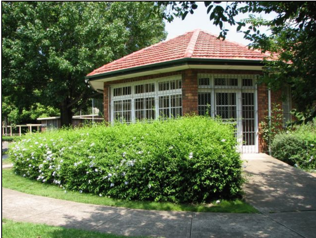
Photo 5: Existing baby health clinic proposed to be relocated to an off-site location and the building demolished to make way for the new children's playground.
