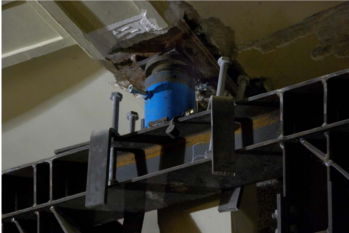
Truss and Jack supporting Centennial Hall
