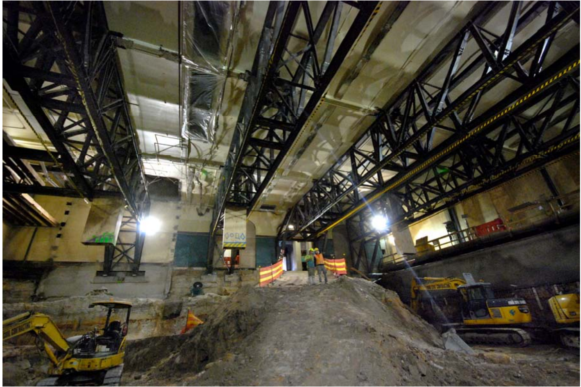
Looking up from base of Excavation
