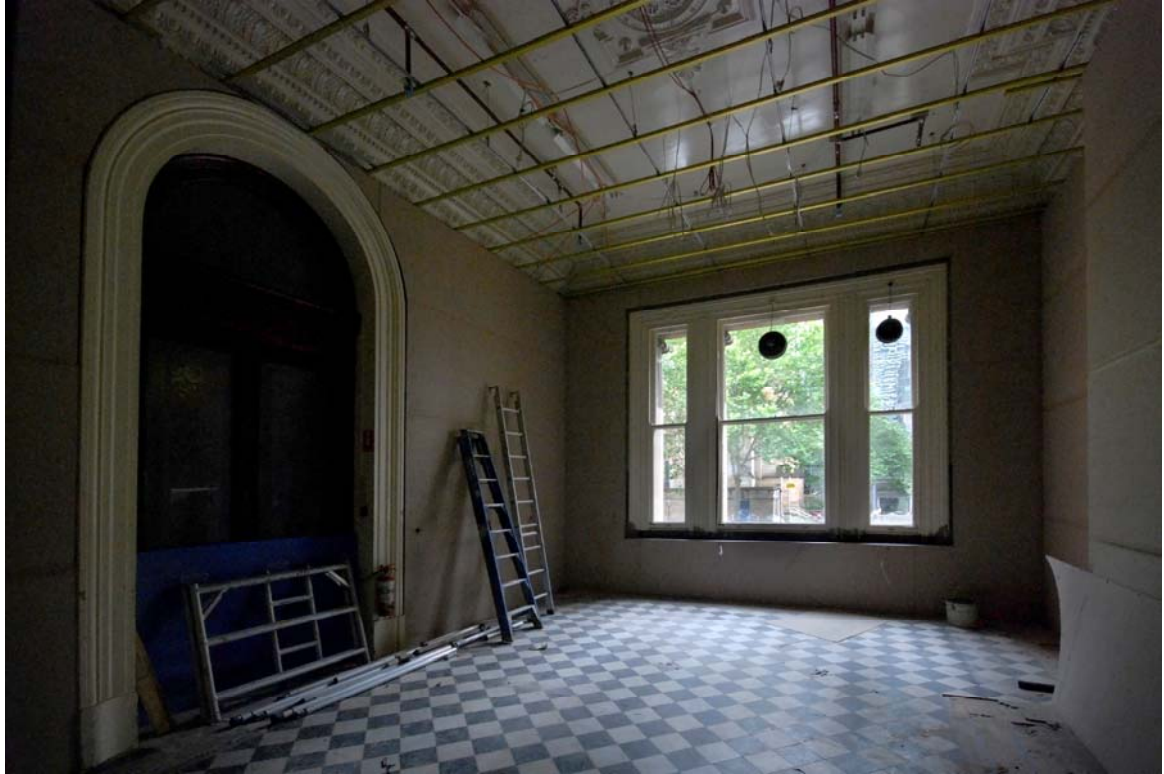
New Kitchen to Centennial Hall Being framed up
