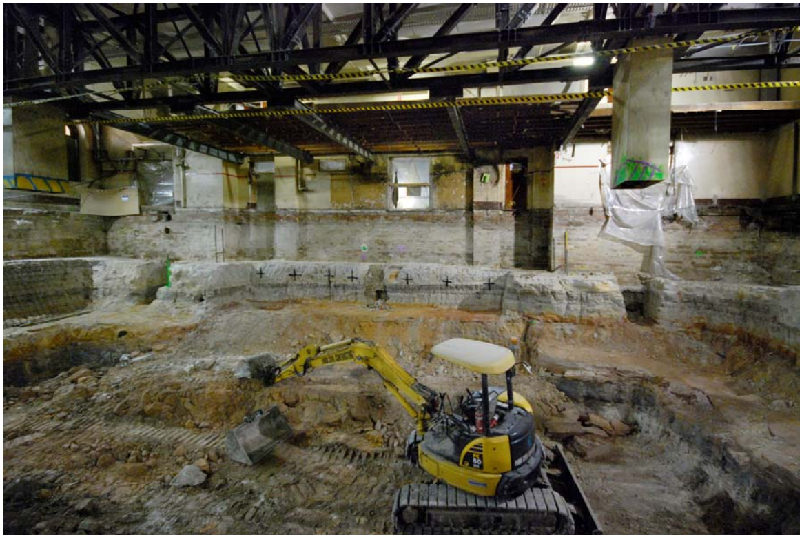
Basement Excavation nearing completion
