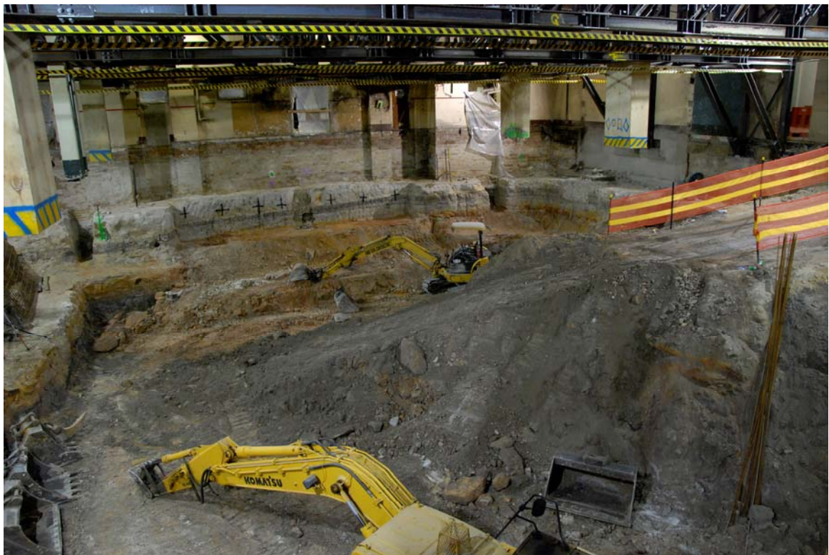
Basement Excavation showing Excavators
