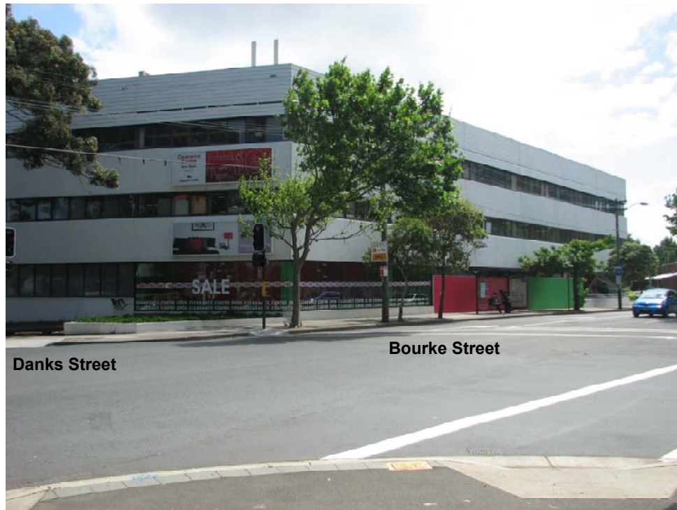
Figure 3: Southeast elevation at the corner of Bourke and Danks Streets
