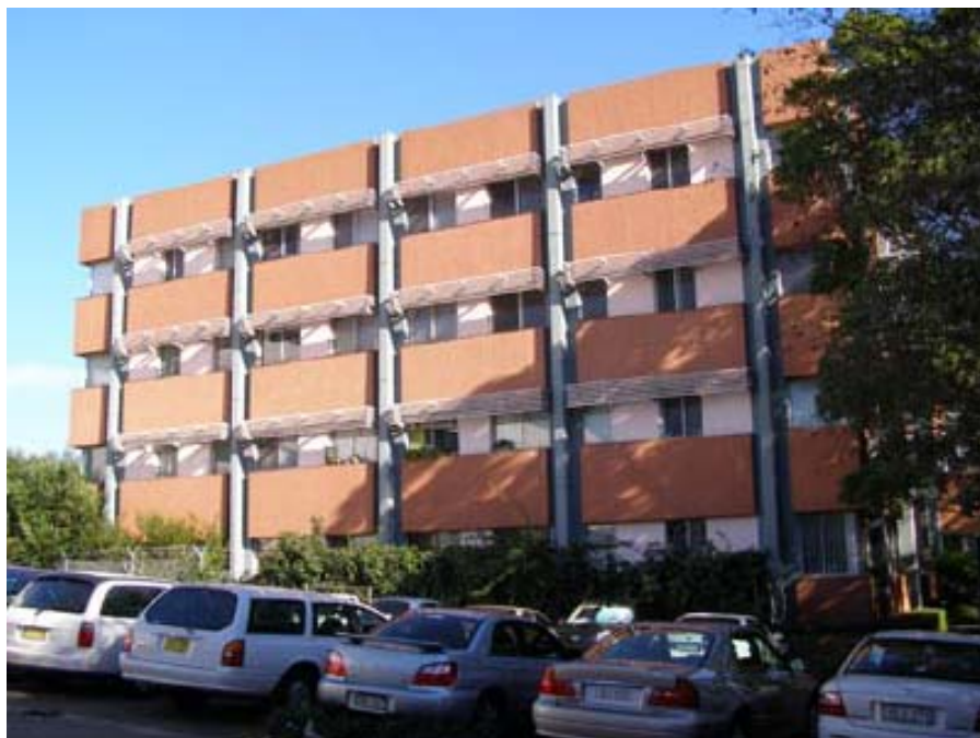
Figure 6: Side elevation of neighbouring Phillip Street residential building
