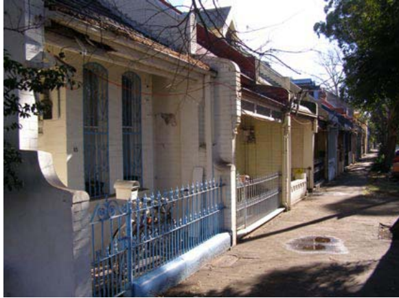
Figure 7: Typical terraces to the north.
