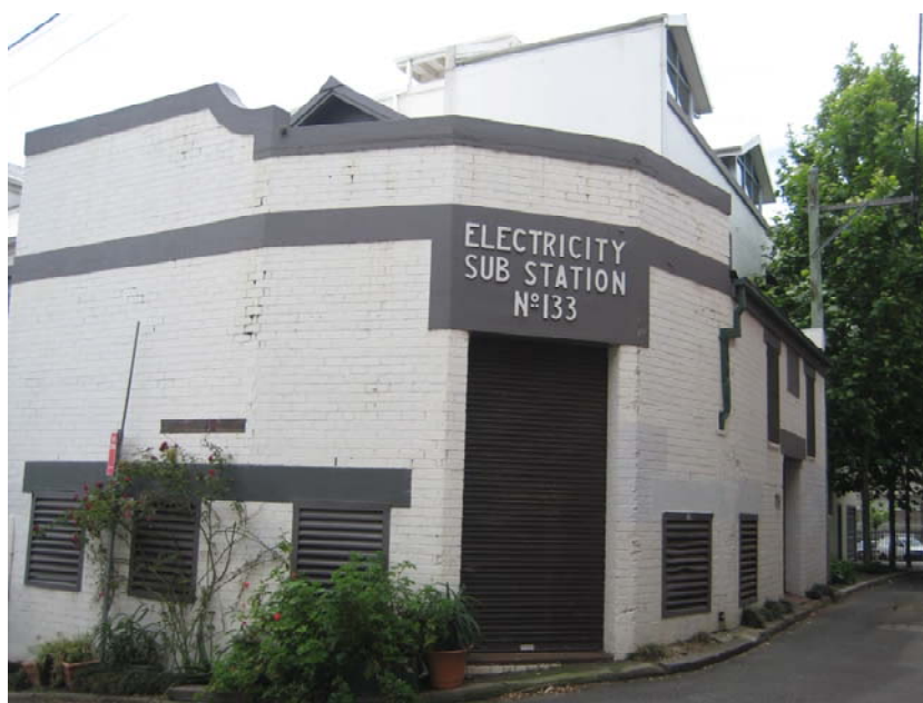
Figure 6: The single storey electricity substation located on the north western corner of Goodchap and Little Riley Streets.
