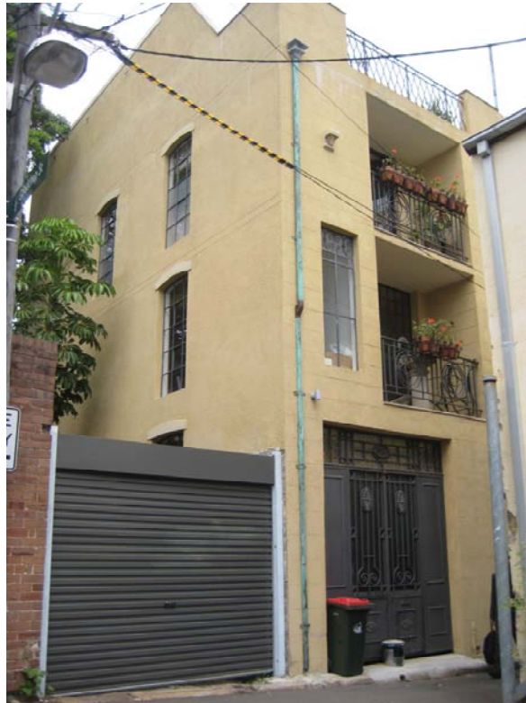
Figure 4: View of 16a Little Riley Street (the neighbouring property to the south), showing the habitable room windows on the north facade.
