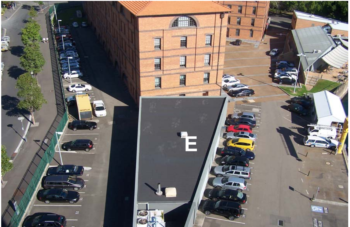
Figure 6 – Building E to be demolished (Building A & B in background)
