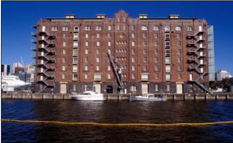
Figure 4 - Building C viewed from water (heritage listed)
