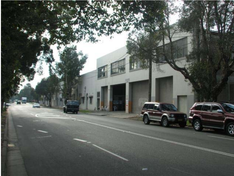
Figure 4 – View looking north-east down Bourke Road showing existing buildings on site.
