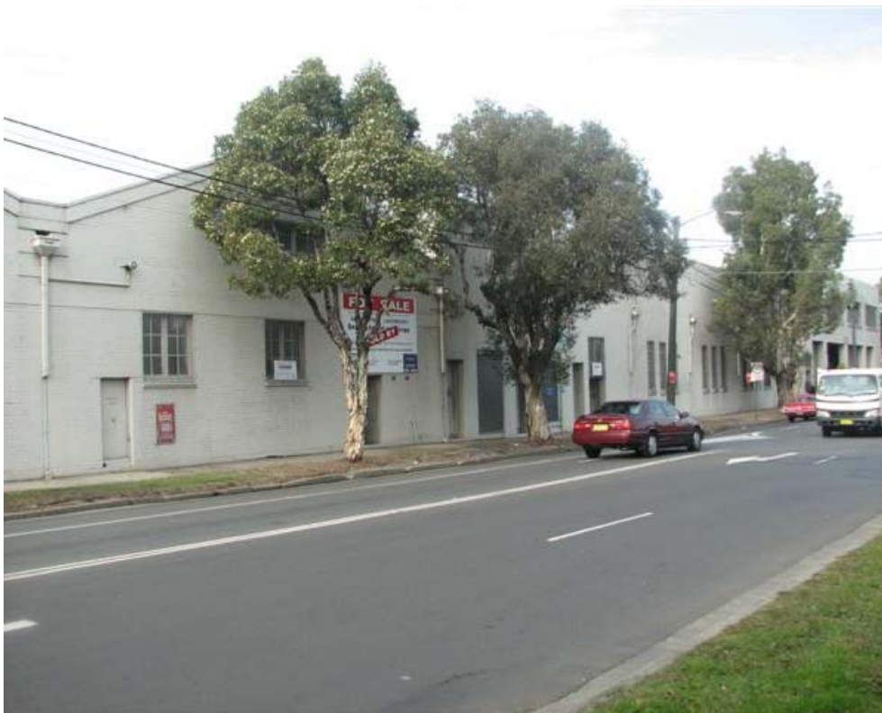
Figure 3 – View looking south-west down Bourke Road showing existing buildings on site.
