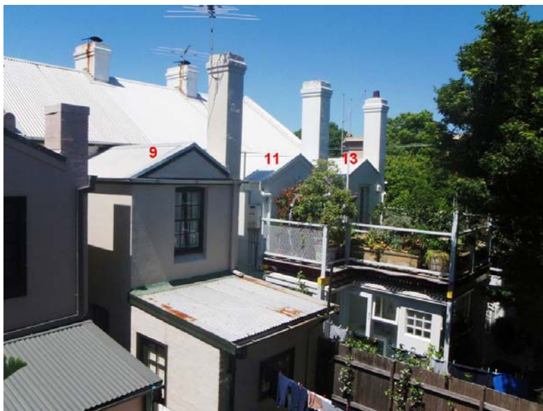
Figure 9 – Rear of Nos. 9 – 13 St Johns Road, taken from the second storey deck of subject site.
