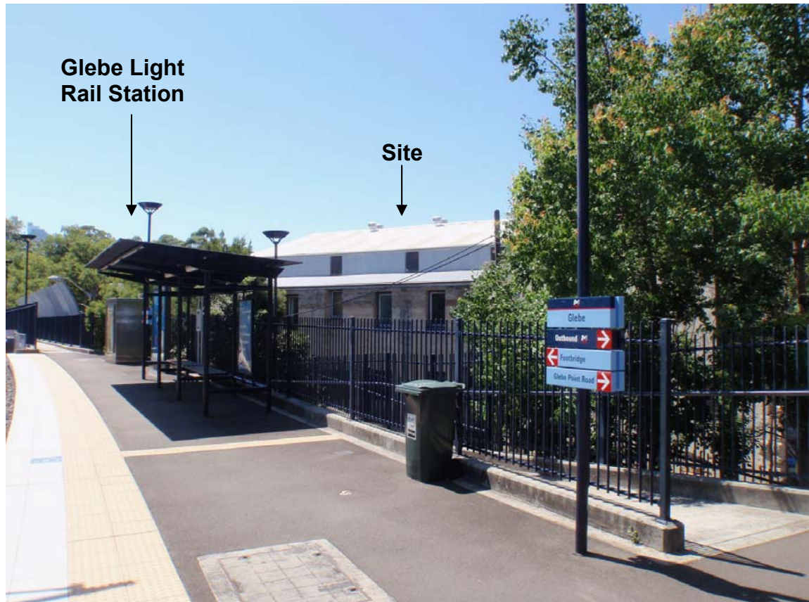
Photo 3: Site directly adjoins Glebe Light Rail Station
