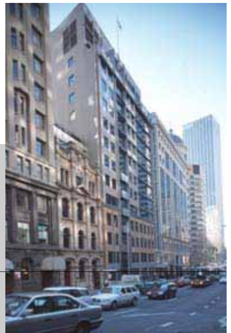
Statement of Heritage Impact - a study and analysis of the heritage significance of any items or site in the vicinity is required
