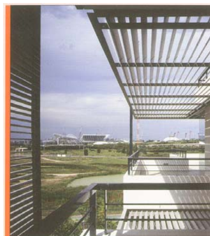
03.37. A combination of louvres provides shading for different times of the day.
