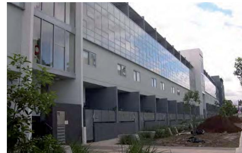
New residential development on Euston Road/McEvoy Street utilises the entry areas of individual units to deal with the level change required due to flooding issues, has no setbacks and directly accesses off Euston Road and should be encouraged..
