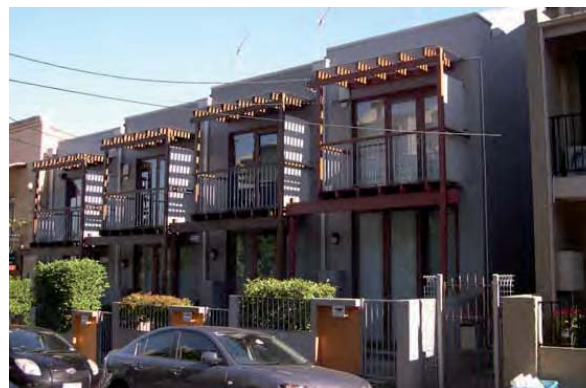
A good example of contemporary terrace dwellings, in keeping with the bulk and scale of traditional terraces in the area, with modelling of the facade to break down flat planes. A strong sense of street address is created with individual entries and low height front fences that delineate between the public and private domain.
