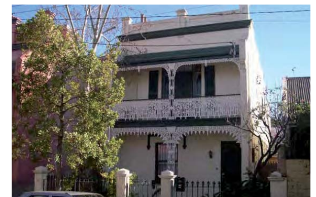
Grand free-standing terrace house is characteristic of the built form in the area and adds to the overall heritage streetscape character.
