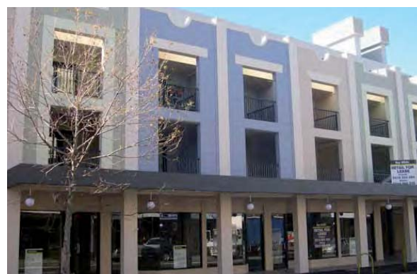
Contemporary example of shop-top housing. Ground floor commercial/retail provides an active street front while the continuous awning provides pedestrian amenity. However, colonnades are not characteristic of King Street, and facade proportions exaggerate the vertical compared to traditional shop front bays and windows.
