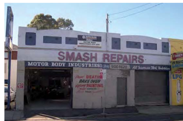
Example of a traditional low scale warehouse found along King Street.
