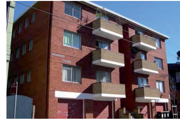
Iredale Street: a 4 storey (3 storey + parking level) residential flat building. Usually this would be considered out of character with the predominant low scale terrace built form but in this location on the edge of King Street it is the garages which are the issue.
