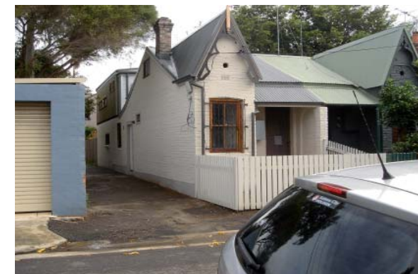
George Street: a good example of a contemporary rear two storey addition to a 1 storey contributory heritage item (Witches Hat houses). The single storey streetscape is retained while the rear addition is clearly delineated from the original house.
