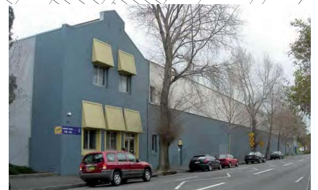
Large areas of blank facades are characteristic of 'big box' industrial buildings. Future mixed use residential development should provide a more active street address through individual street entries, windows and balconies opening onto the street.
