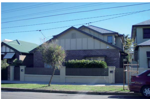
Sympathetic unobtrusive rear addition to a 1 storey Federation semi enables retention of 1 storey streetscape character.
