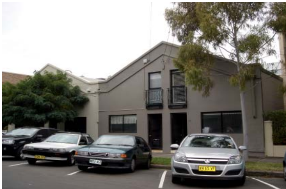
Adaptive re-use of warehouse buildings is characteristic of this precinct and should be encouraged.
