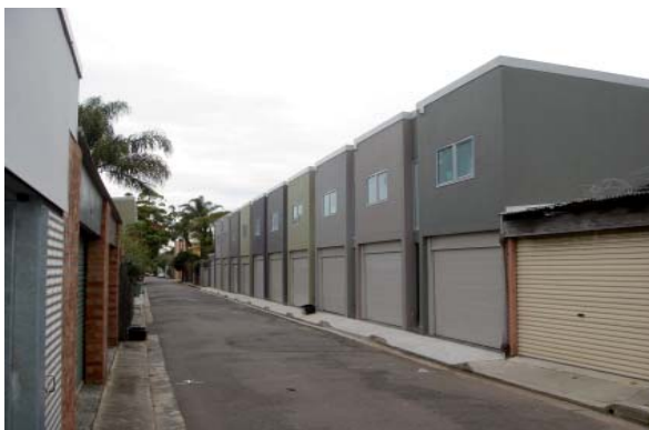
Belmont Lane— unsympathetic garage/studio developments on laneways. Potential improvements would be to setback the second storey to create a balcony space and introduce a pitched roof form which would reduce the overall bulky appearance.
