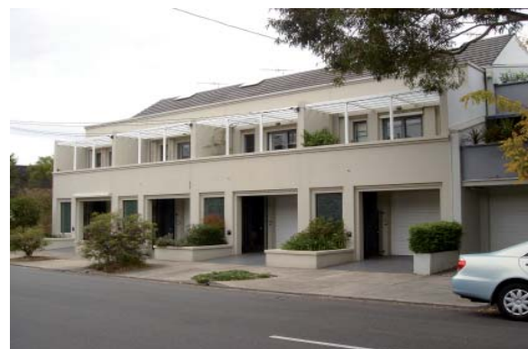
Garages on the street frontage (whilst they are recessed) are not in keeping with the streetscape character and resemble more of a laneway character.
