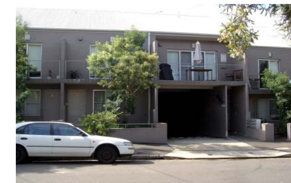
Figure 4.2.3.1: Townhouse on Burren Street, Erskineville
