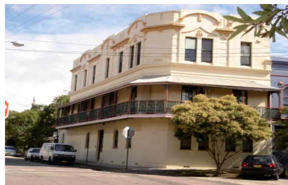
Figure 4.2.8.1: Former corner commercial building on Albert Street, Erskineville
