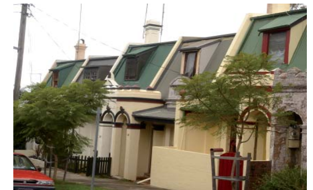
Figure 4.2.4.3: Dormer style terrace on Gibbes Street, Newtown
