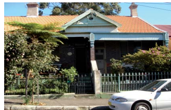
Figure 4.2.2.2: Semi on Union Street, Erskineville
