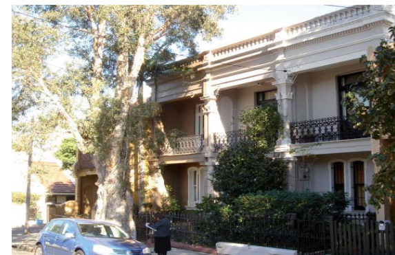
Figure 4.2.4.2: Parapet roof terrace on Malcolm Street, Erskineville
