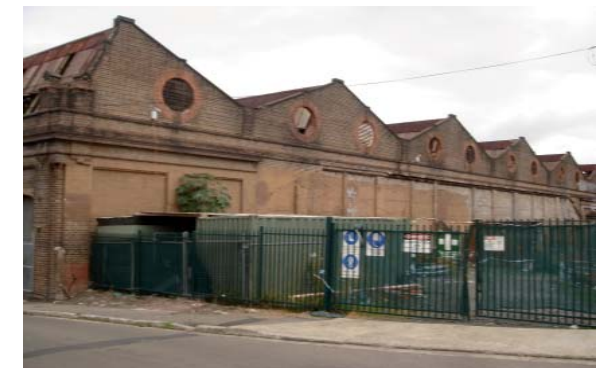
Figure 4.2.10.1: Tram sheds on Angel Street, Newtown
