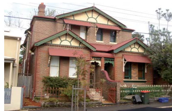
Figure 4.2.2.1: Semi on Macdonald Street, Erskineville
