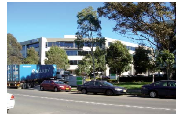
Figure 4.2.12.1: Euston Road commercial building
