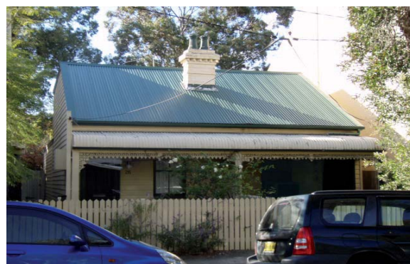
Figure 4.2.1.2: Timber cottage on Phillips Street, Alexandria
