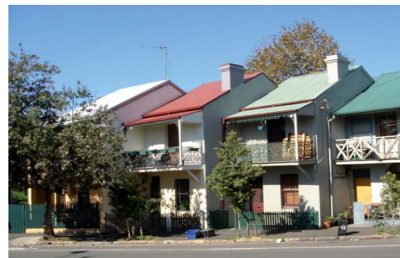
Figure 4.2.4.1: Pitched roof terrace on Henderson Road, Alexandria
