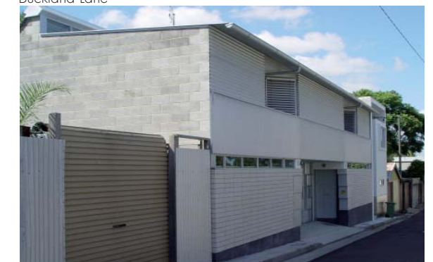
Figure 4.2.13.2: Modern laneway development on Brandling Lane
