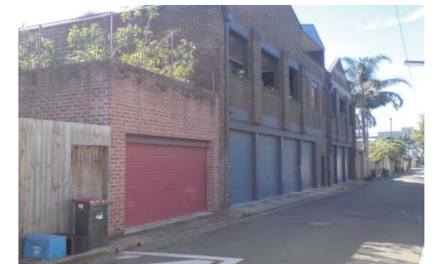
Figure 4.2.13.1: Older style development builds on laneway on Buckland Lane
