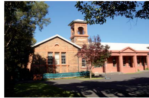
Figure 4.2.14.2: Erskineville primary school
