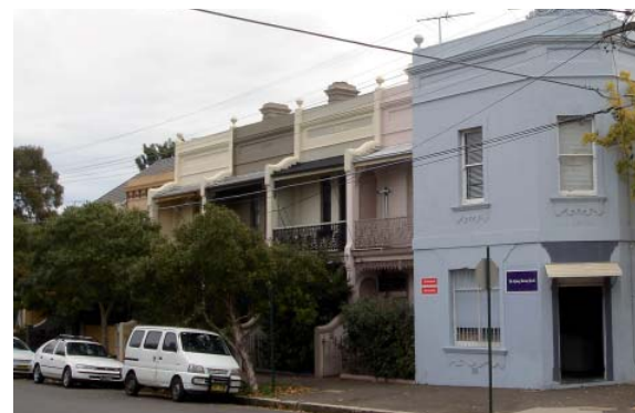
Figure 4.2.4.4: Balcony set between fin walls on Belmont Street, Alexandria
