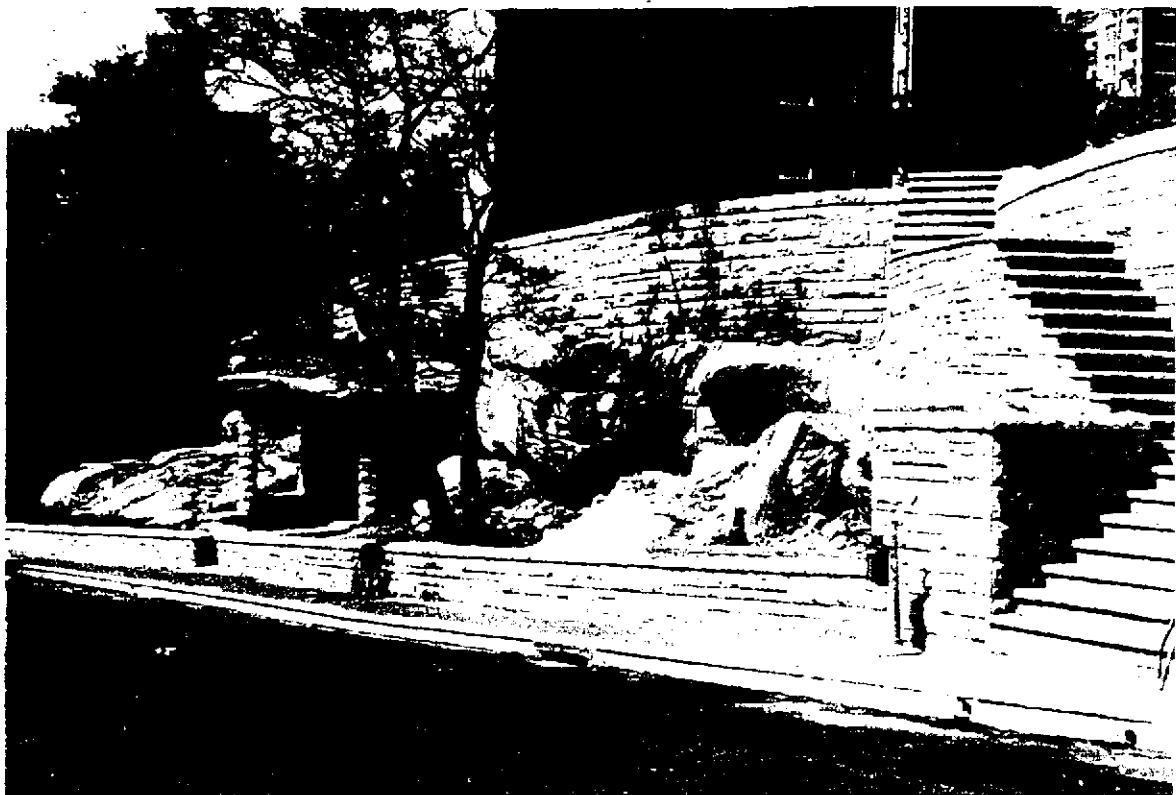
Fig. 22 The south-eastern corner of McElhone Reserve c. 1953, showing the full extent of the large retaining wall built on top of the main rock bench and the formalised treatment of the natural cave/grotto on Billyard Avenue. The retaining wall is said to be on the same alignment as the one built for Alexander Macleay in the late 1820s. Photo: courtesy Mrs. Sylvia Berzins.
