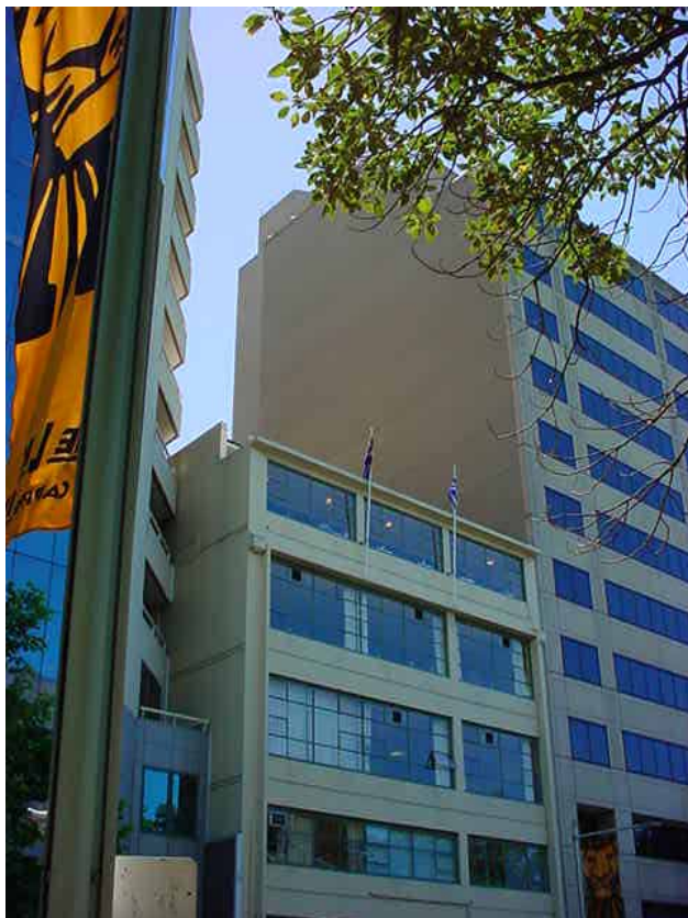
Hellenic Club Building, illustrating height of adjoining property to the north at 231-249 Elizabeth Street
