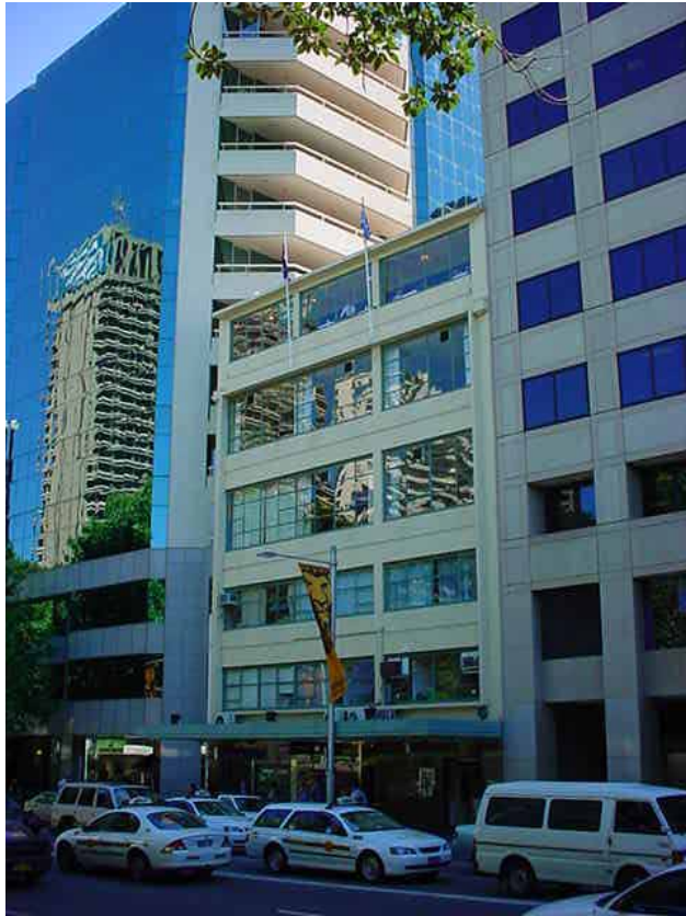
Hellenic Club Building, illustrating height of adjoining property to the south at 255-269 Elizabeth Street
