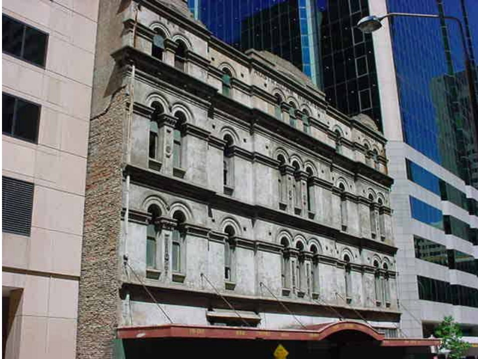
Façade of the AWU Building, fronting onto Castlereagh Street
