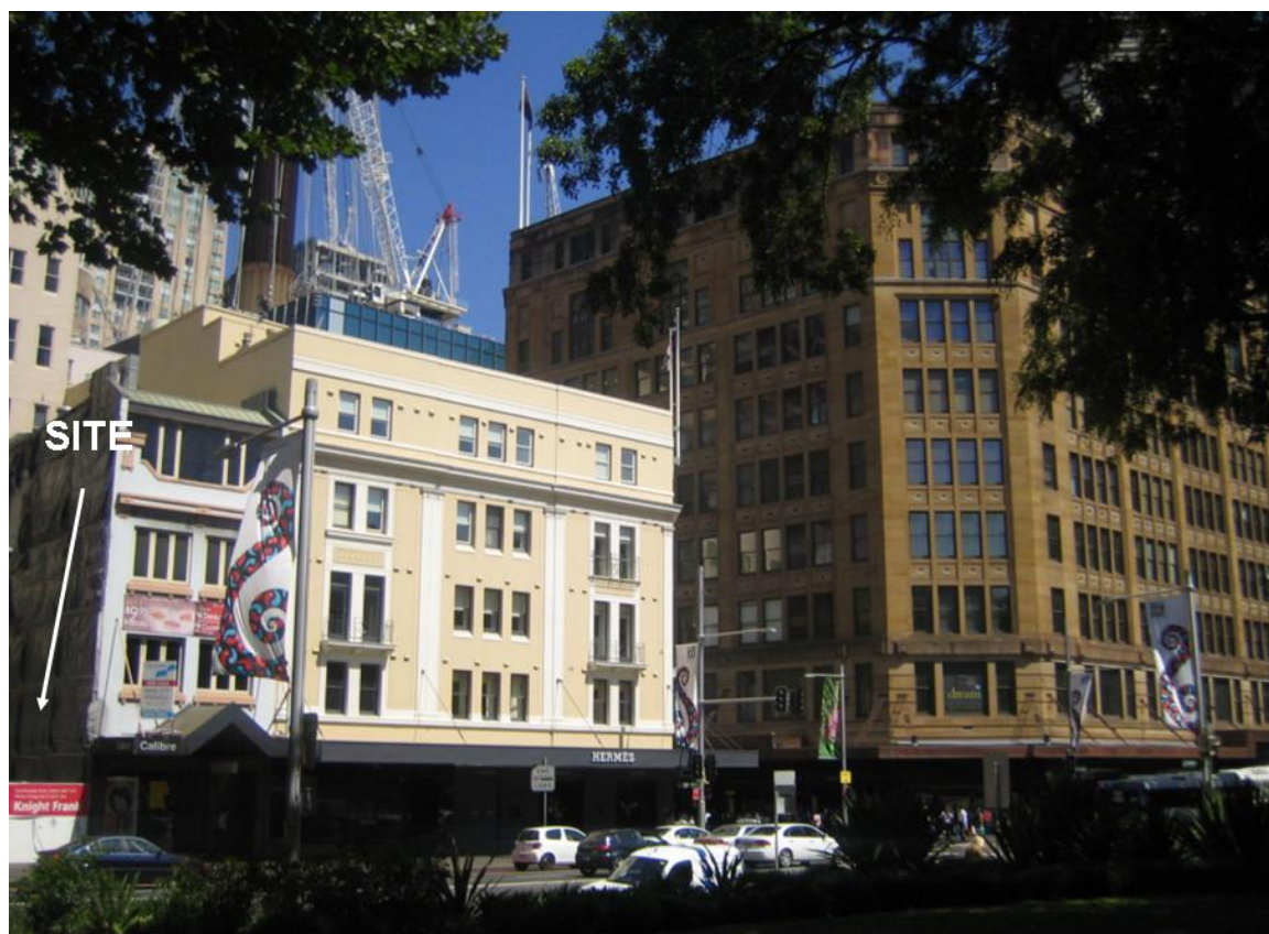
Figure 4: Existing development to the north of the site
