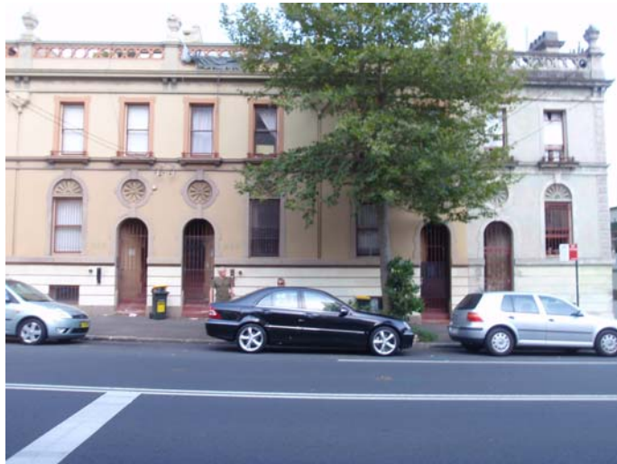
Photo 8: Bourke Street elevation of terrace row
