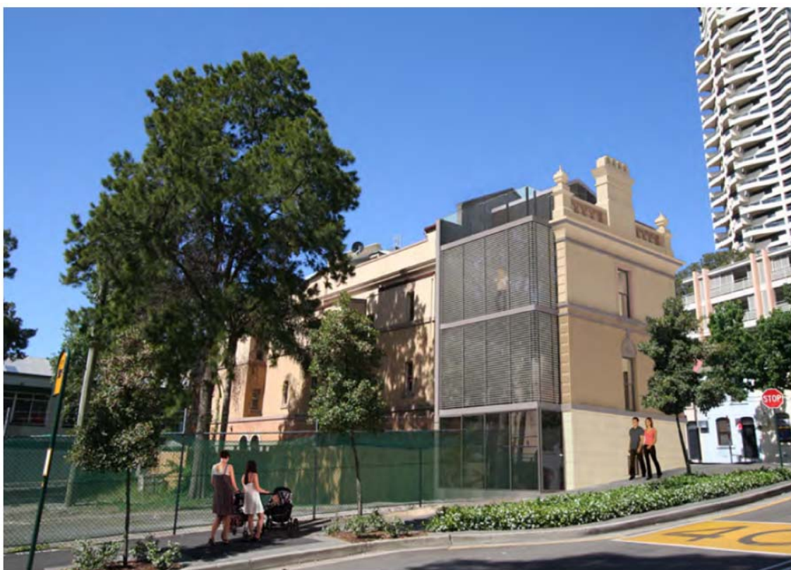
Figure 3: Photomontage of western elevation. Note that this depicts the original design; the current design lowers the height of this elevation and removes the horizontal string course to improve its relationship with the remainder of the row
