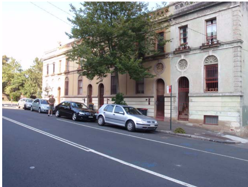
Photo 7: Bourke Street elevation of terrace row
