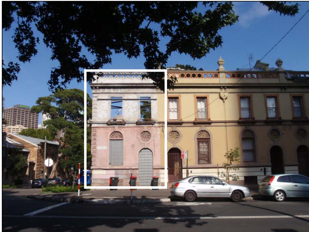
Photo 1: Subject site – outlined as seen from Bourke Street
