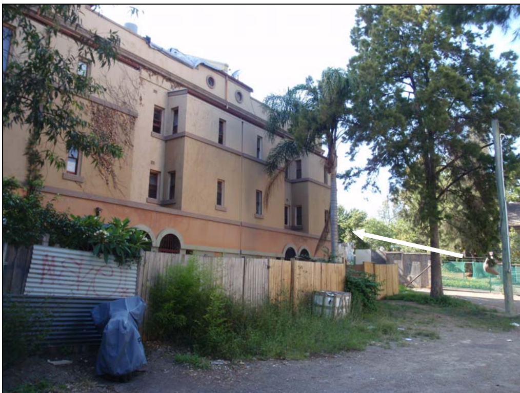
Photo 5: Rear of the row of terraces. Rear of the subject site is not visible but the location is indicated by an arrow
