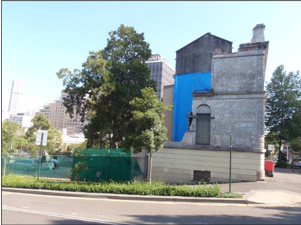
Photo 2: Side of subject site – showing damaged facade to Stanley Street
