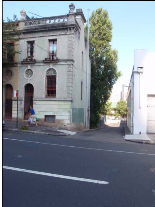
Photo 6: Bookend terrace at the opposite end of the row of terraces to the subject site
