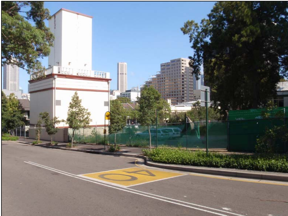
Photo 4: RTA tunnel exhaust stack building and vacant RTA land to the rear of the subject site
