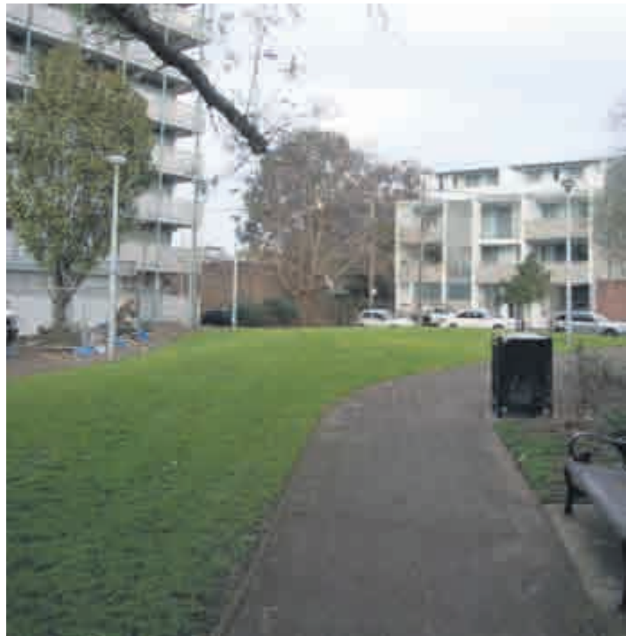
The park in Camperdown earmarked for Sydney's first Common Ground housing project
