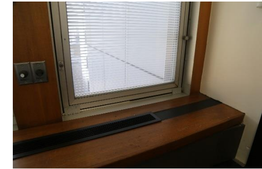
2018 Registers with original/early details and in-operational regulator switches
