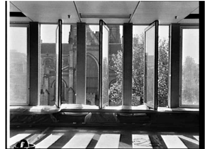
1968 Photograph showing the double-glazed pivot windows
