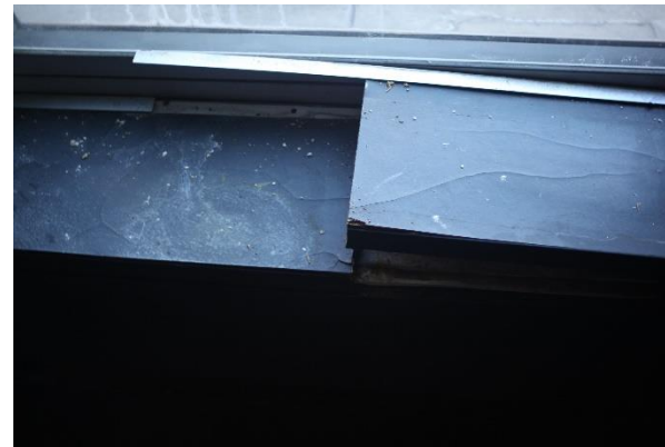
2019 removed register replaced with pre-cast concrete and reclad (Level 3)
