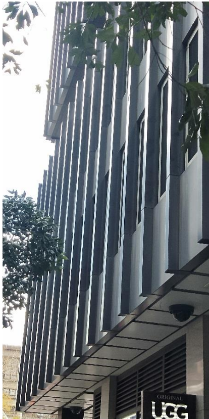
Fig 20. New cladding to exterior (Source: Extent)
