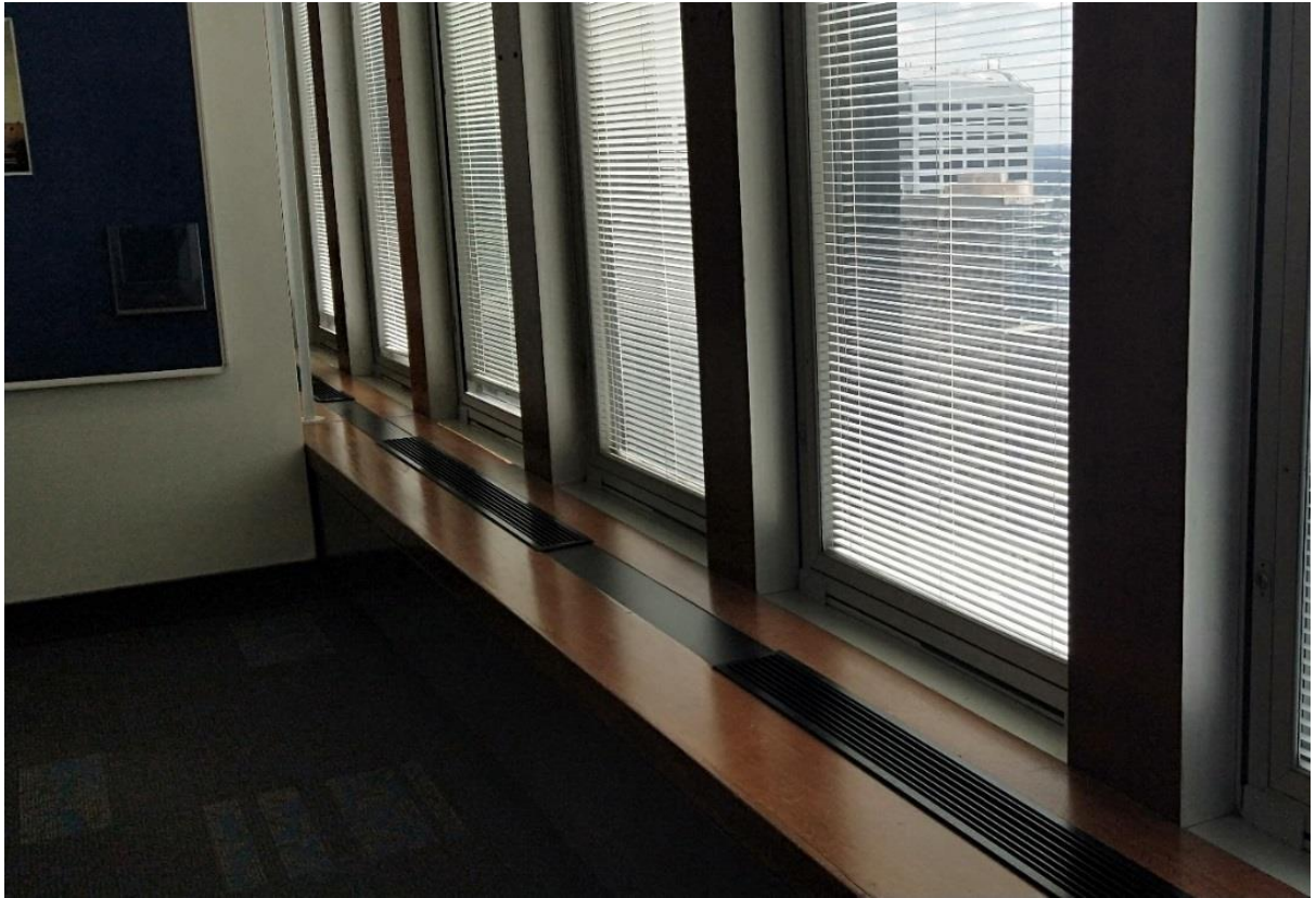
Fig 17. Interior of the building showing the original air conditioning vents (Source: Extent)
