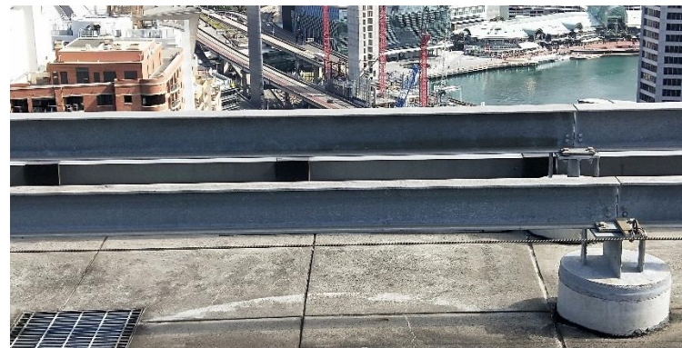
2018 Overclad façade detail as seen from roof – covering granite capping
