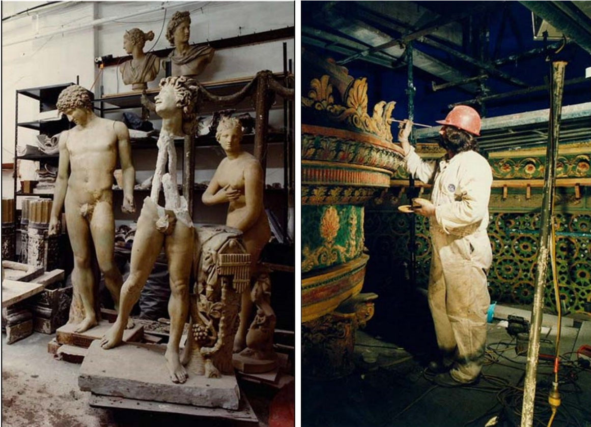
Figure 225 – Restoration work in progress at Capitol Theatre. One left: statues were repaired and recast based on replicas from other theatres (1994). On right: an artist at work during restoration (1994).
