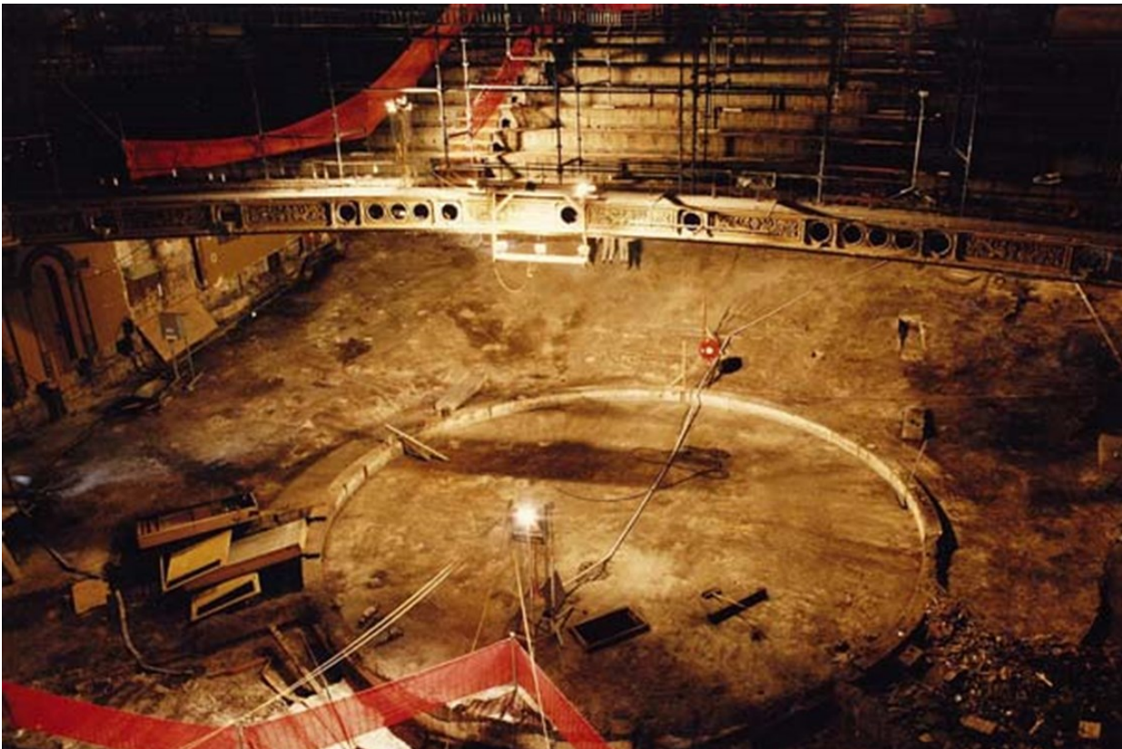
Figure 240 – Concrete tank, otherwise known as the seal pit uncovered during the restoration of the Capitol Theatre, 1994.
