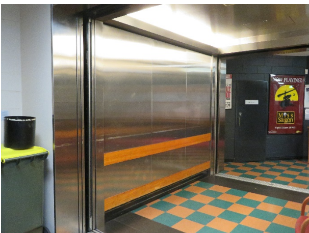
Figure 141 – Goods lift in Back of House area.
