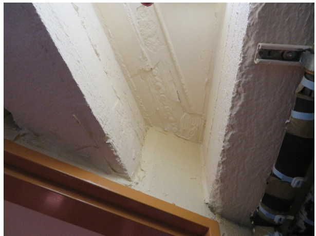
Figure 125 – Ceiling in kitchenette with remnants of pressed metal.
