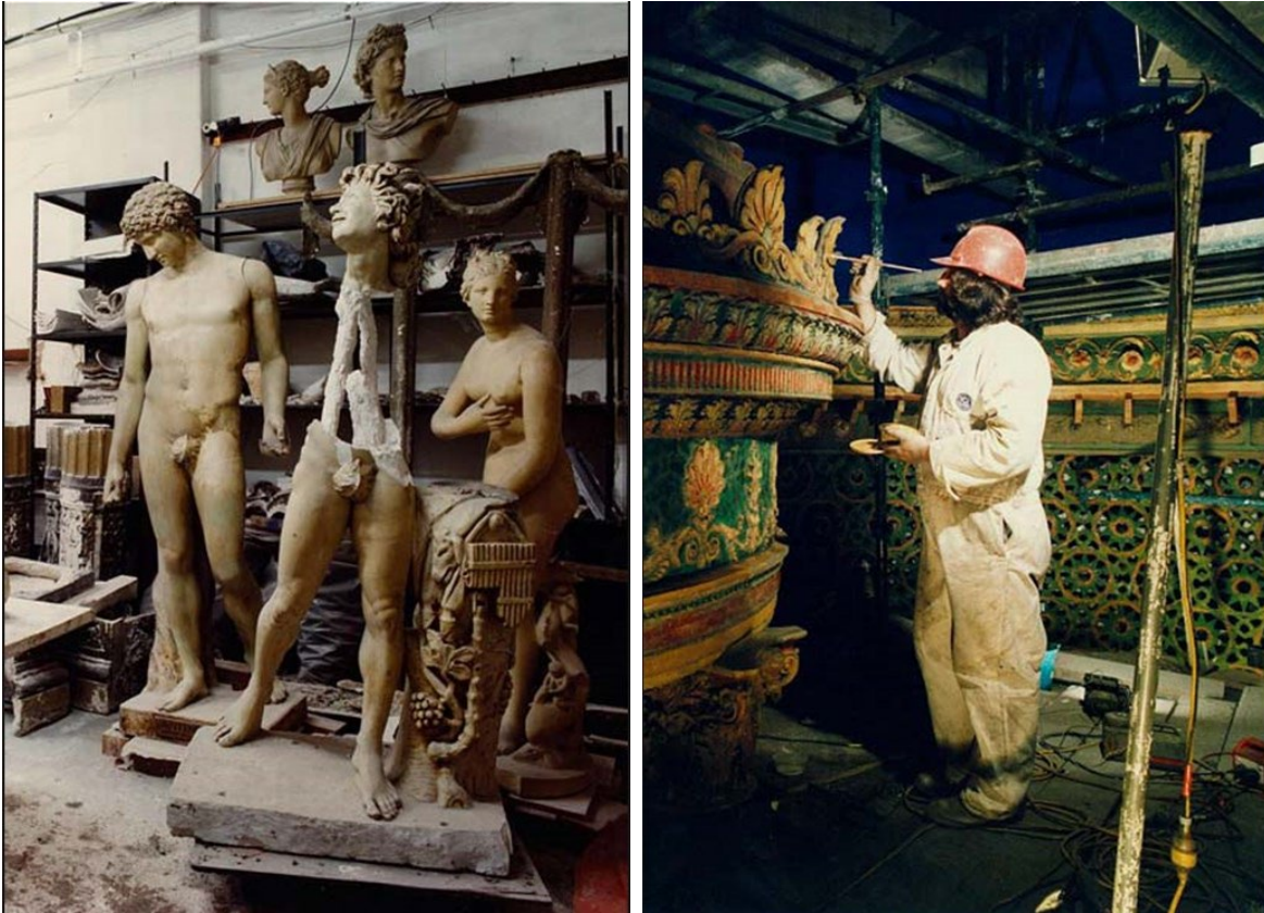
Figure 208 – Restoration work in progress at Capitol Theatre. One left: statues were repaired and recast based on replicas from other theatres (1994). On right: an artist at work during restoration (1994).
