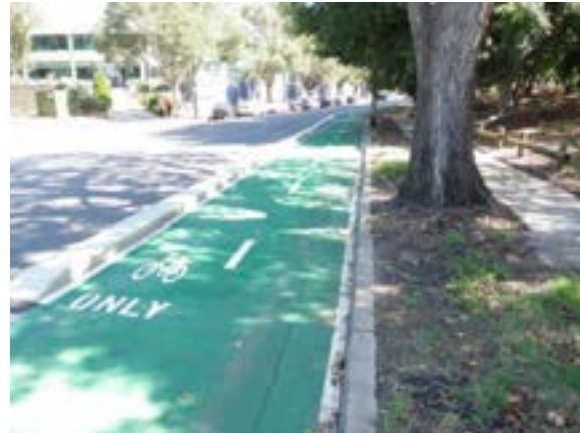
Figure 2.3: Bourke Road Separated Cycleway
