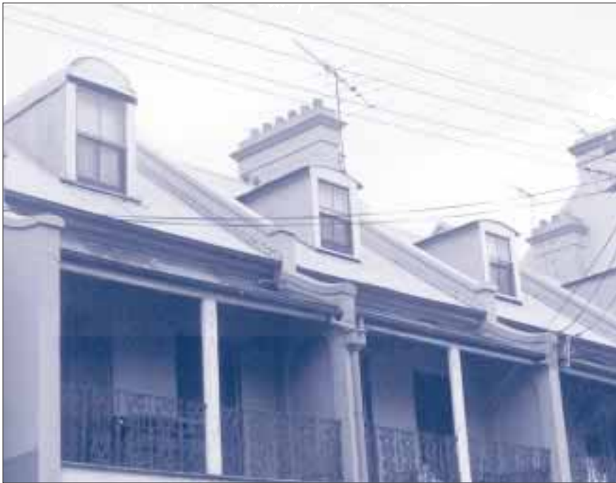
Original dormer window (left). New dormers in this row have been designed to reflect the character of the original dormer, while clearly being new work
