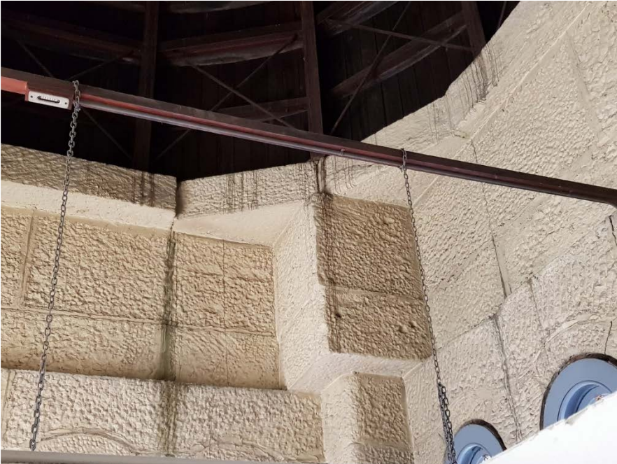
Figure 37: Water Staining From Dome Roof
