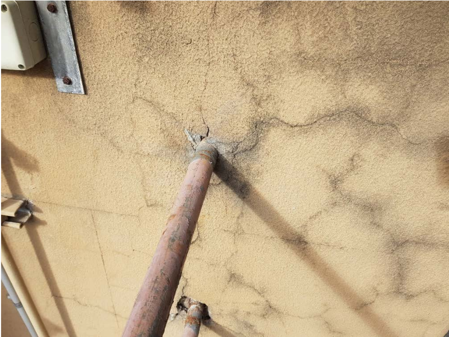
Figure 9: Cracking Around Embedded Railing
