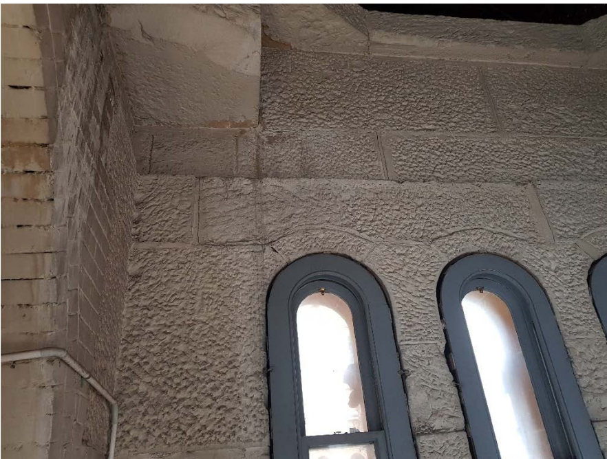
Figure 14: Diagonal Cracking Through Bed Joints Above Windows
