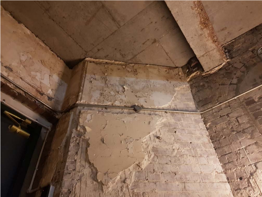
Figure 41: South Fire Escape Damp and Spalling Concrete
