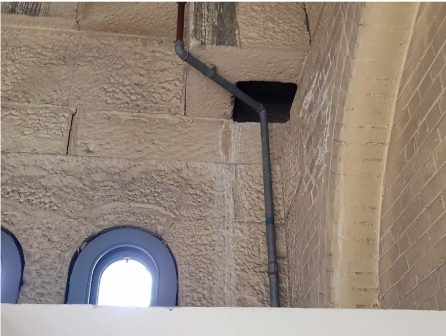
Figure 36: Water Staining From Dome Roof
