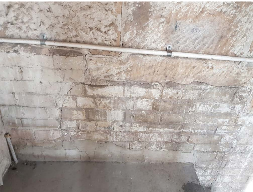
Figure 18: Vertical Cracking at Sandstone Brick Interface
