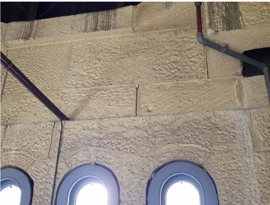
Figure 16: Diagonal Cracking Through Bed Joints Above Windows
