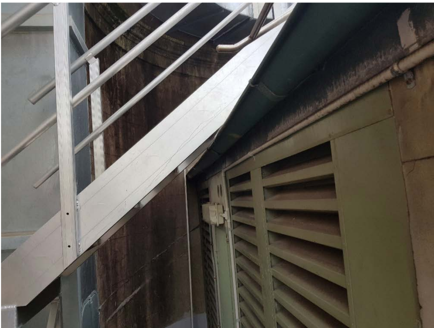
Figure 50: Bowing Gutter Above North West Flat Roof
