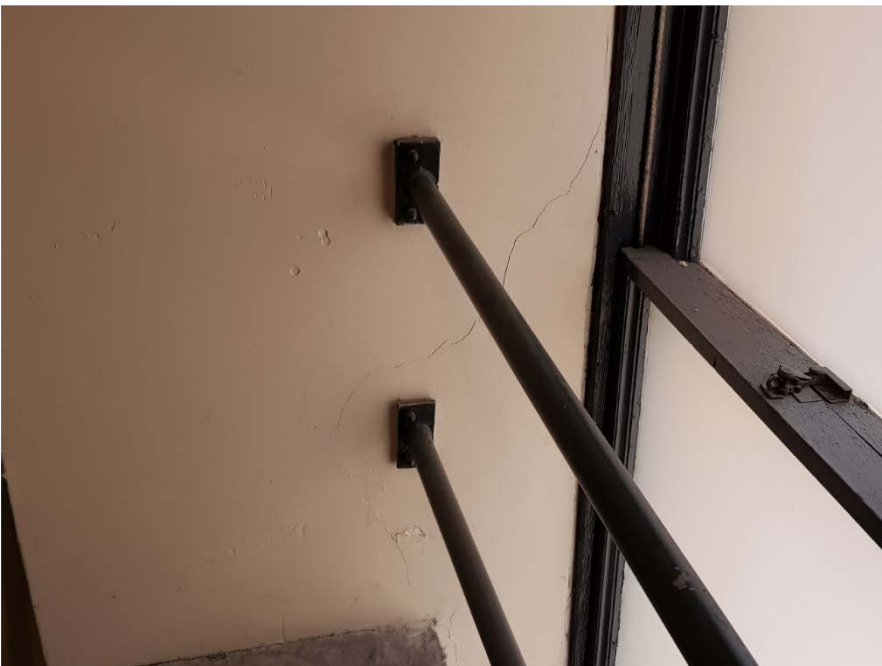
Figure 20: Cracking Around Railing Fixings
