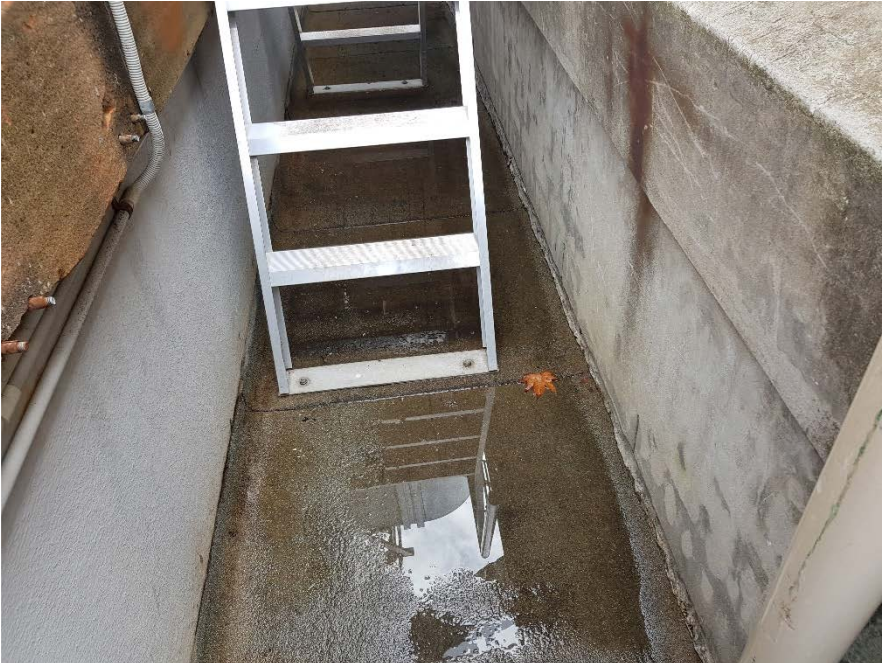
Figure 33: Ponding Water on North East Flat Roof
