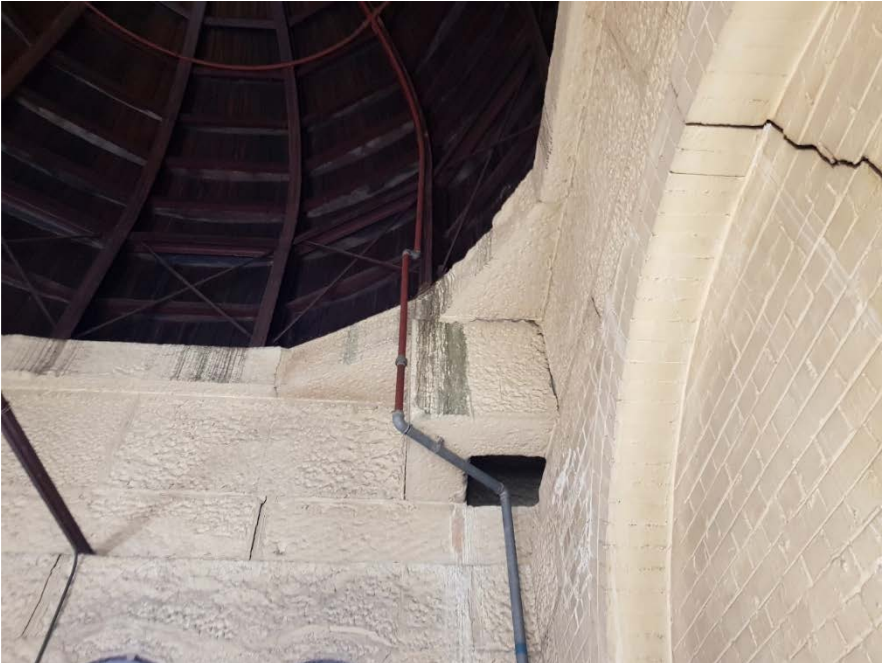
Figure 35: Water Staining From Dome Roof
