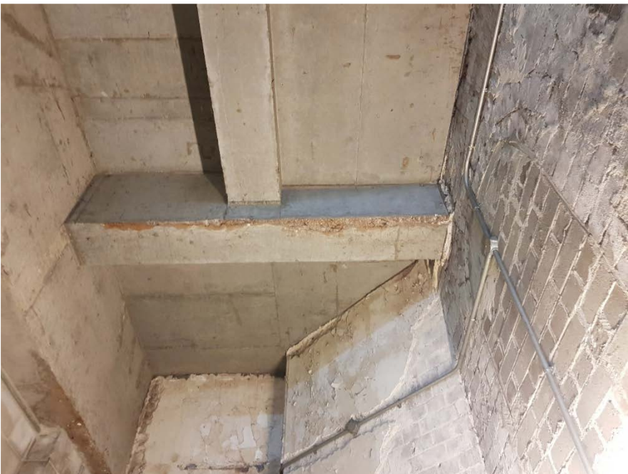
Figure 42: South Fire Escape Damp and Spalling Concrete
