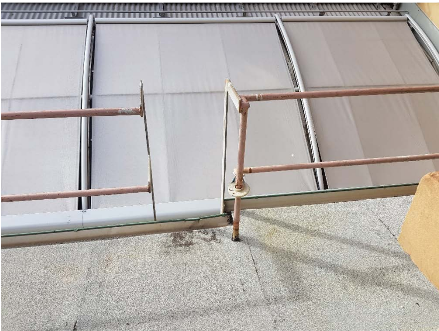
Figure 6: Balustrade North West
