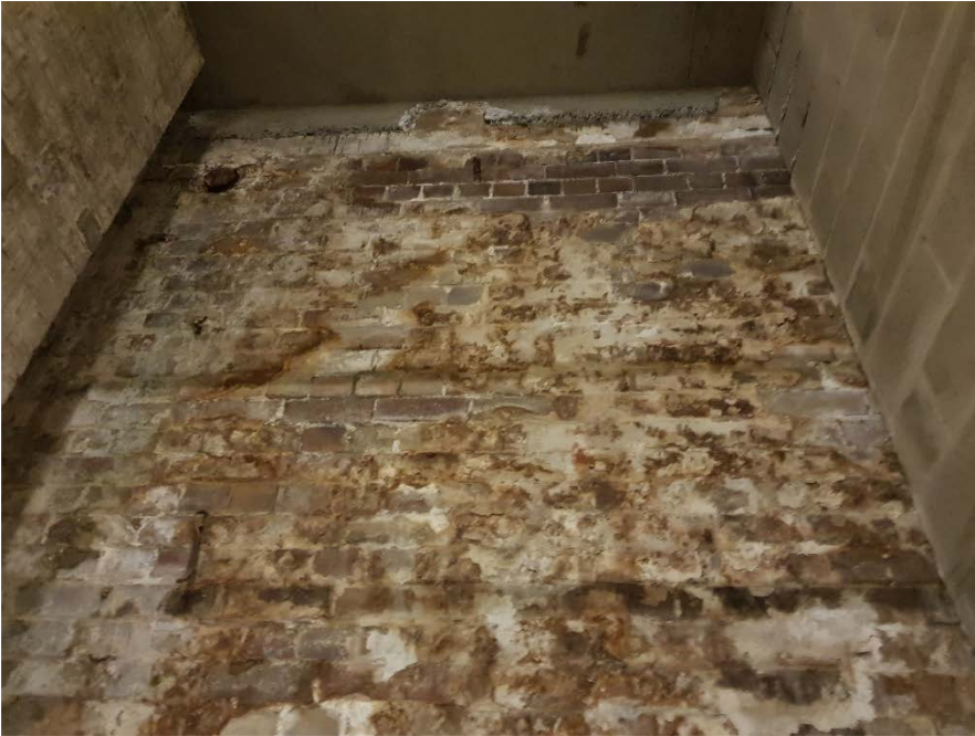
Figure 45: Damp Wall in Lower Ground Fire Escape
