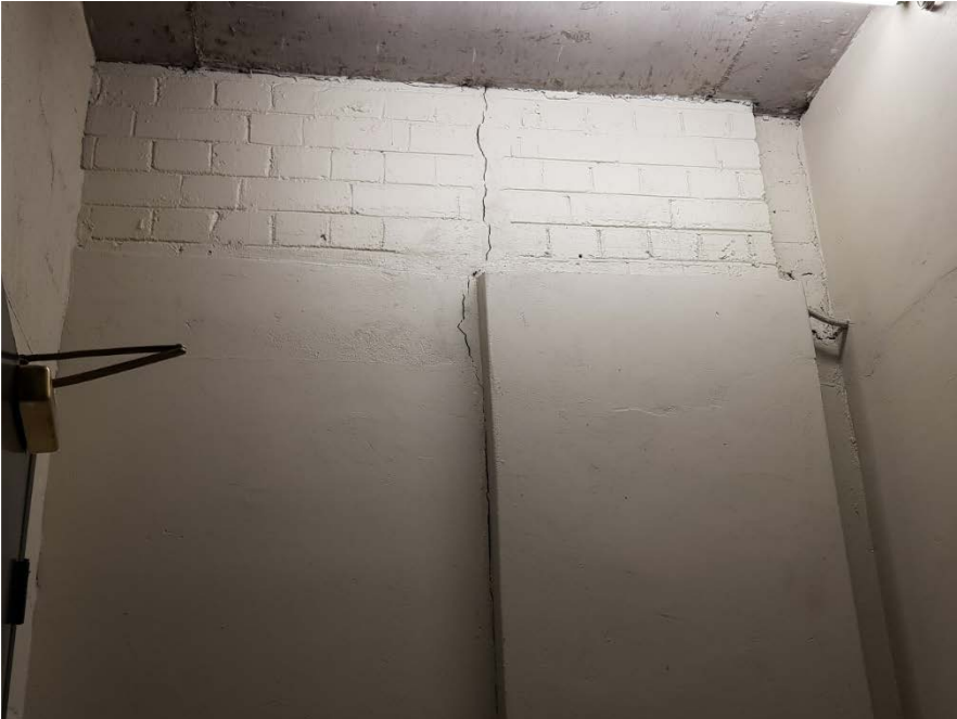
Figure 21: Vertical Cracking in Masonry
