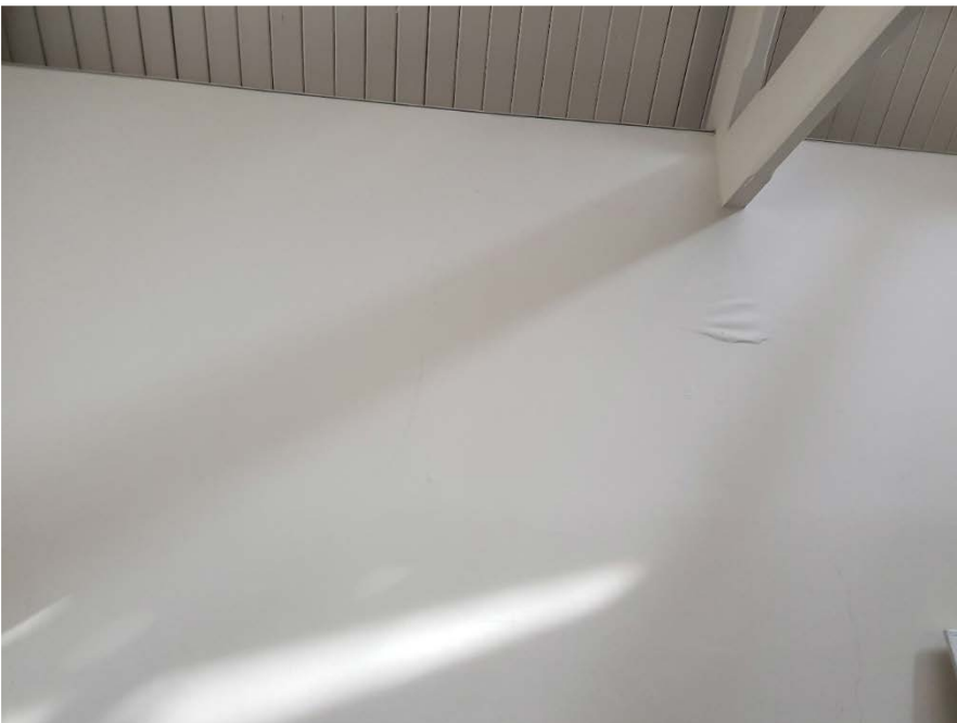
Figure 38: Signs of Water Ingress From The Victoria Room Roof
