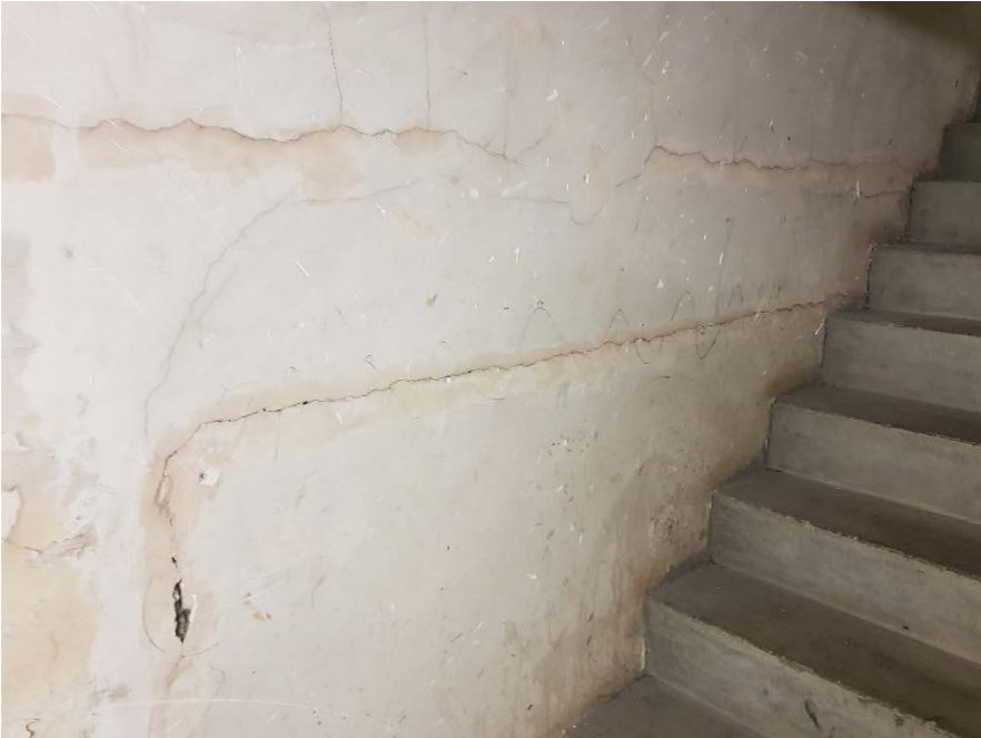
Figure 19: Cracking in Northern Fire Escape Walls
