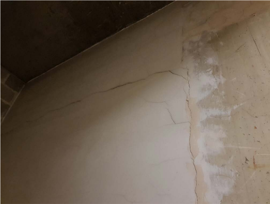
Figure 27: Fire Escape Cracking
