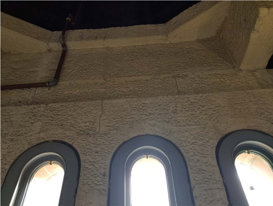
Figure 15: Diagonal Cracking Through Bed Joints Above Windows
