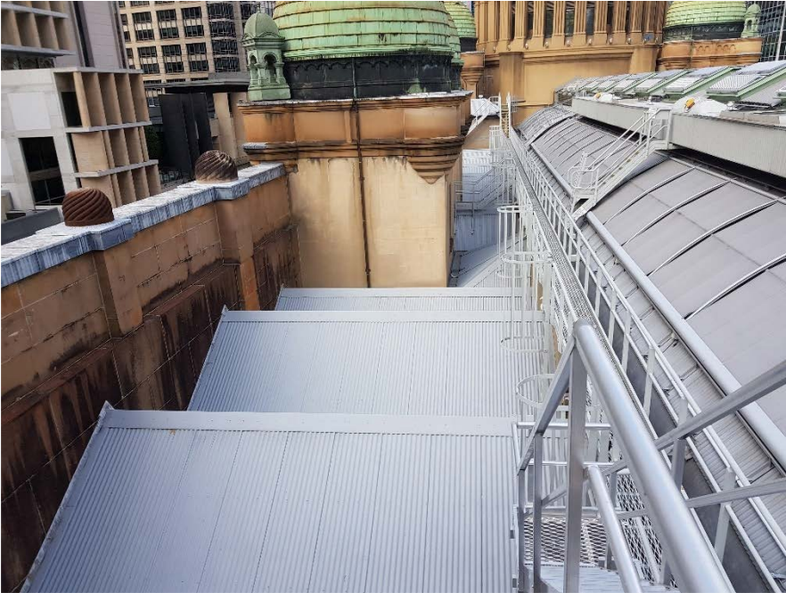
Figure 11: Typical New Access Walkways
