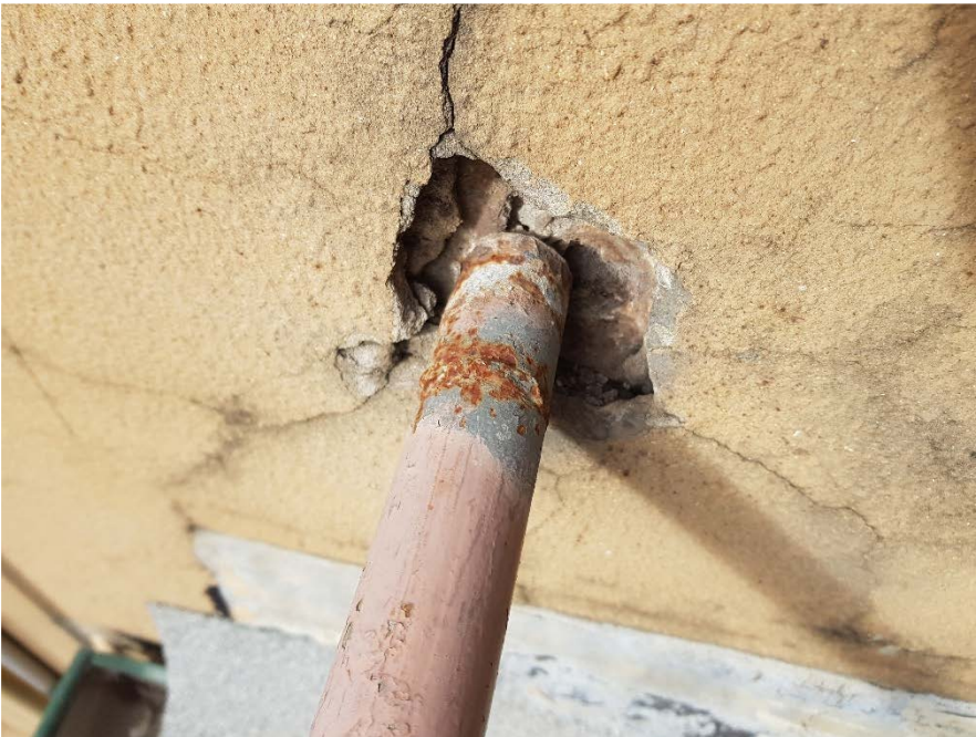
Figure 8: Original Railing Broken Off from Wall
