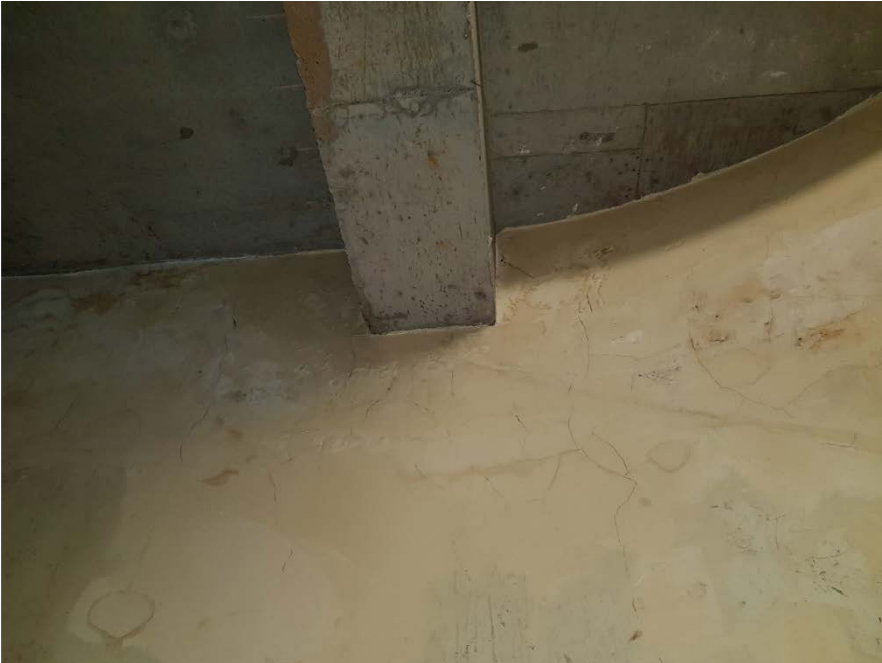
Figure 31: Damp Walls in Fire Escape
