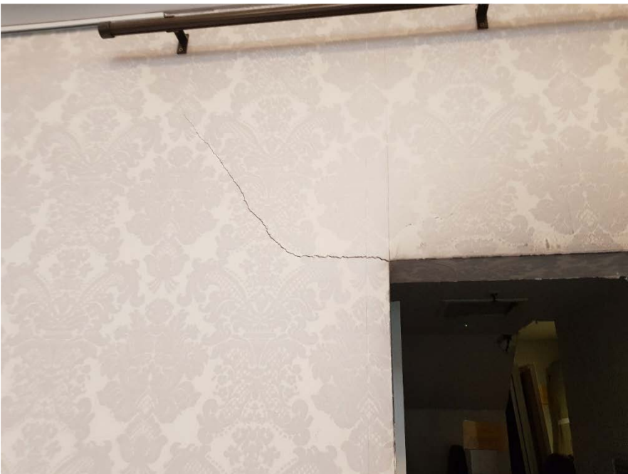
Figure 26: Diagonal Cracking in Tea Room Lintel
