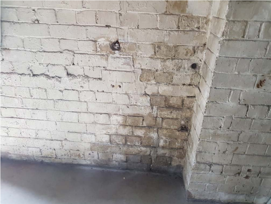
Figure 17: Cracking Around Old Embedded Fixings
