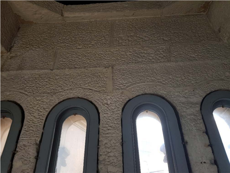
Figure 13: Diagonal Cracking Through Bed Joints Above Windows
