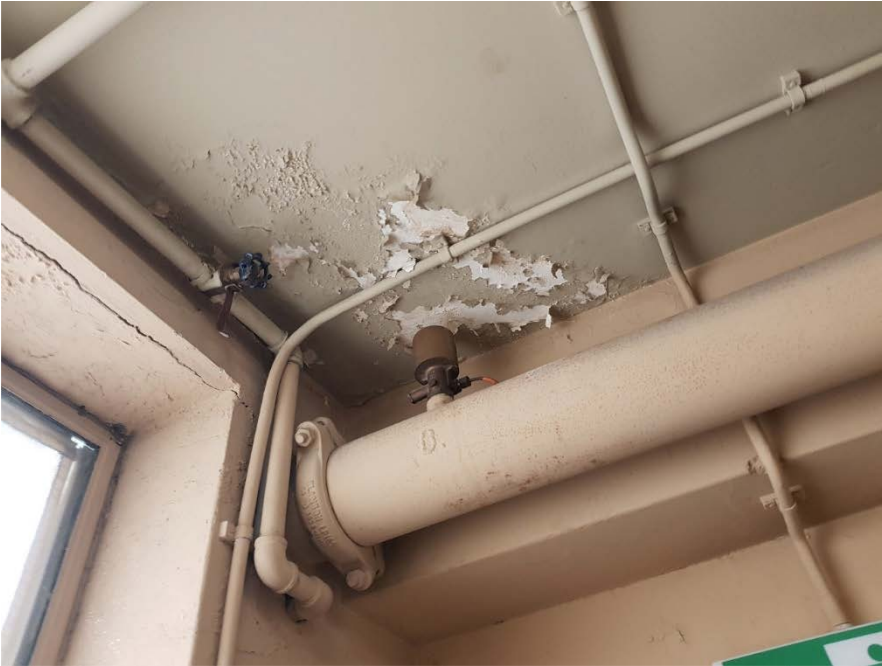
Figure 29: Spalling Concrete
