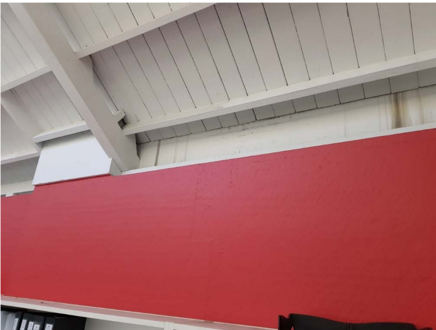
Figure 40: South East Meeting Room Water Staining
