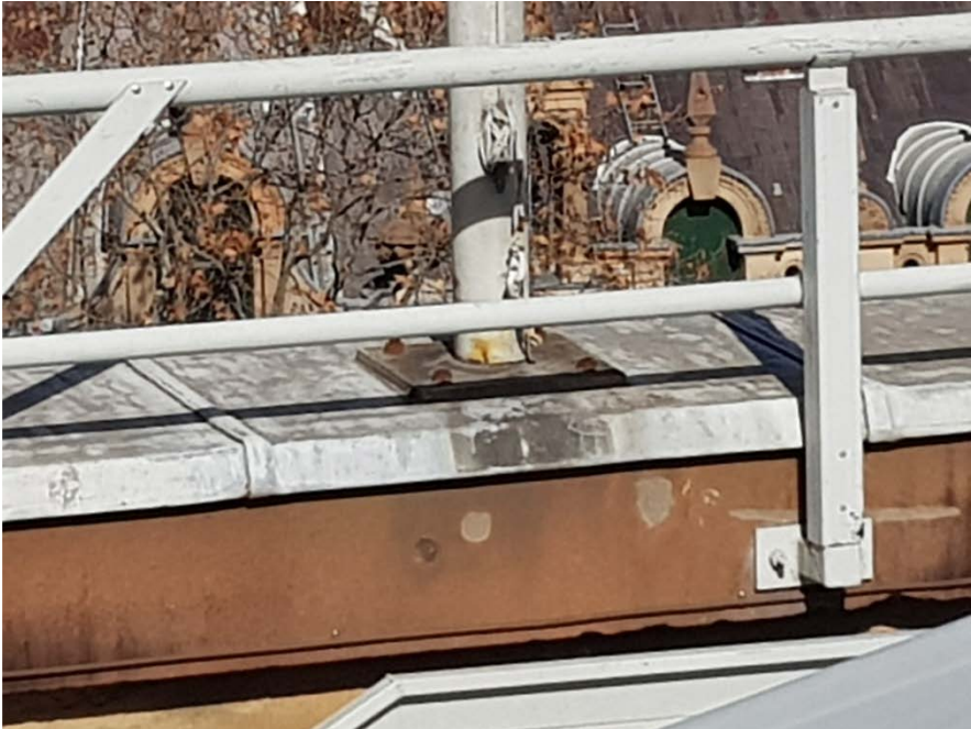
Figure 5: Corroded Flag Pole Connections South End
