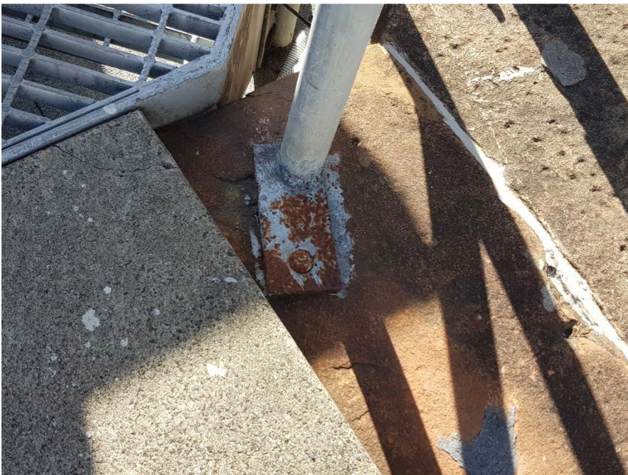
Figure 10: Corroded Connection of Access Structure South End
