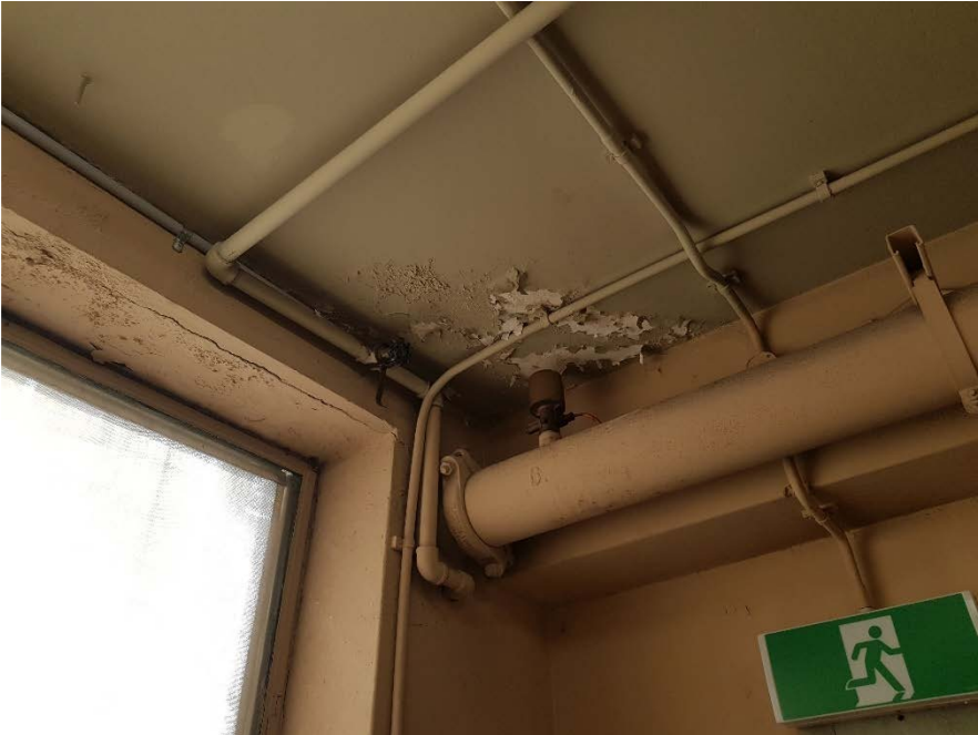
Figure 25: Cracking in Lintel
