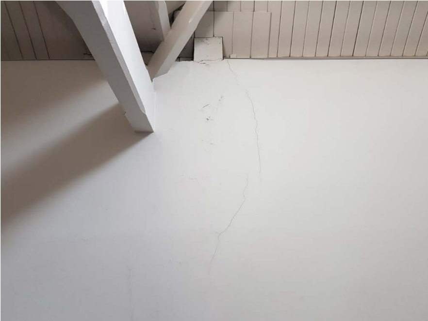
Figure 39: Signs of Water Ingress From The Victoria Room Roof
