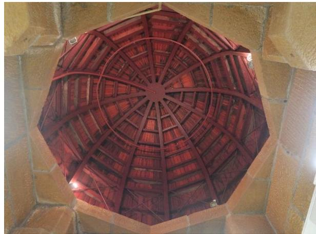
Picture 32 – View up to the timber framing of one of the minor domes
