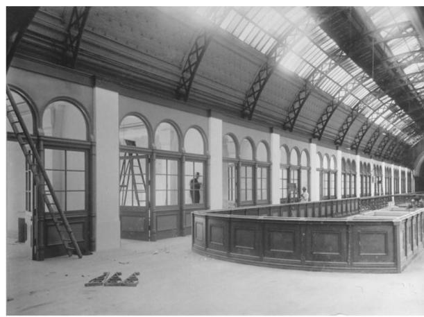
Picture 77 – Balustrades of the upper levels were enclosed with timber cladding, 1918
