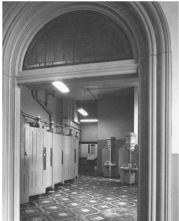
Picture 89 – Some of the men's bathrooms with their cast iron and porcelain urinals and partition posts were amongst the few internal areas to remain moderately intact
