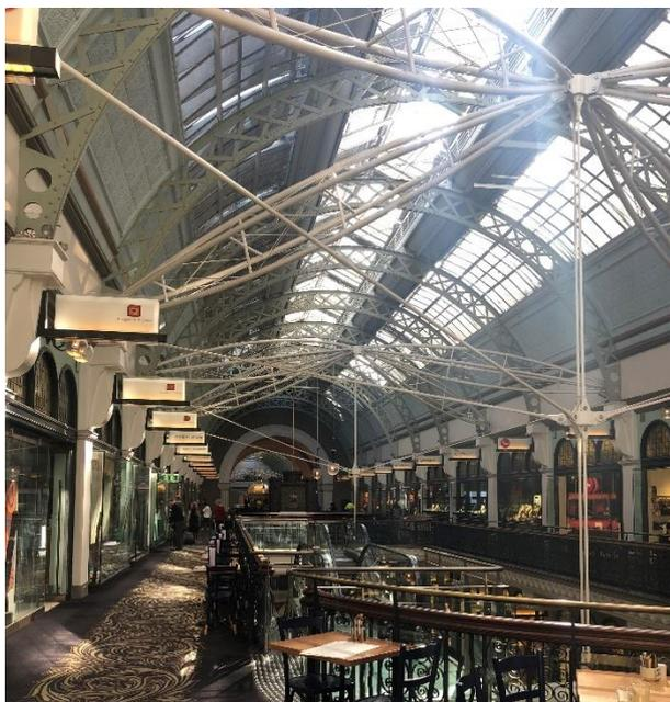
Picture 27 – View of second floor shopfronts, note the steel wishbone structures that the escalators are suspended from
