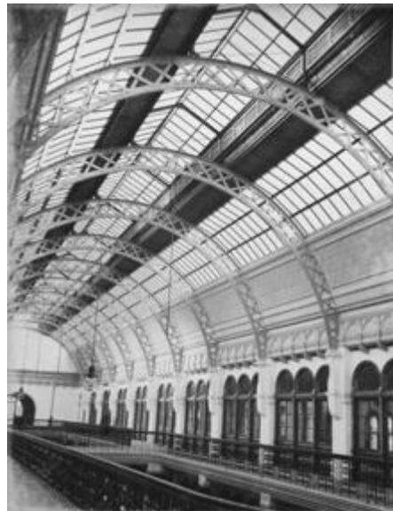
Picture 61 – View of barrel vault roof and shopping gallery, 1898
