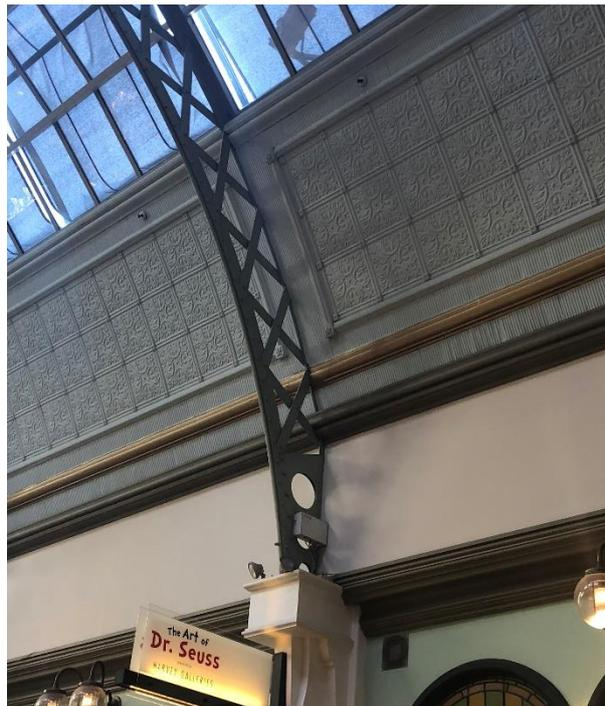
Picture 40 – Pressed metal panels above second floor shopfronts
