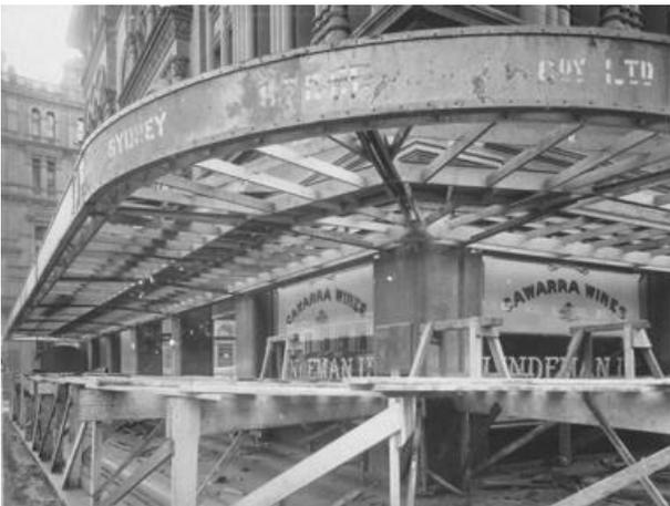
Picture 68 – Construction of the steel cantilevered awning, 1918
