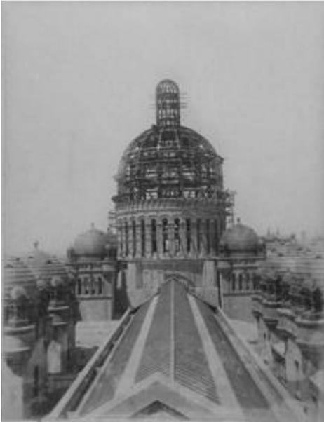
Picture 52 – View of the framing of the central dome, c. 1898
