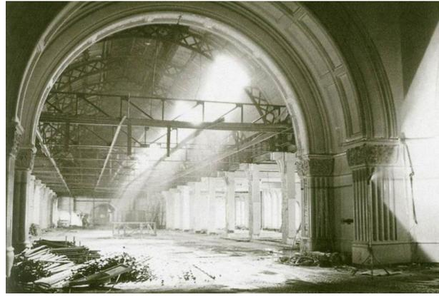
Picture 87 – The top floor at the commencement of works in 1984. The structure which supported the false ceiling under the barrel vault is evident and the concrete infills of the gallery voids had yet to be removed. Sheets of corrugated iron which replaced the original glass had been removed to allow light to be admitted
