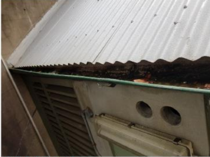
Figure 51: Broken Fixing on Gutter Above North West Flat Roof
