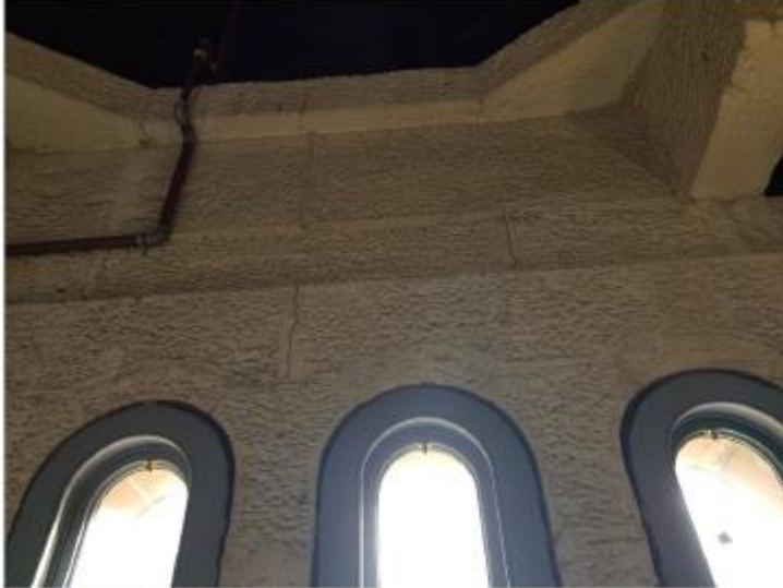
Figure 15: Diagonal Cracking Through Bed Joints Above Windows
