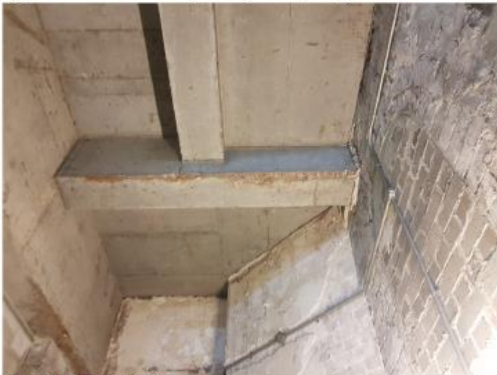
Figure 42: South Fire Escape Damp and Spalling Concrete
