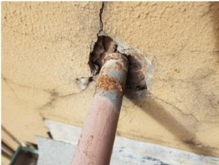
Figure 8: Original Railing Broken Off from Wall
