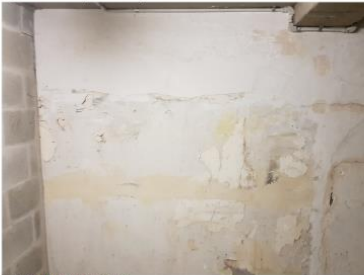
Figure 34: Damp Fire Escape Walls Under North West Flat Roof
