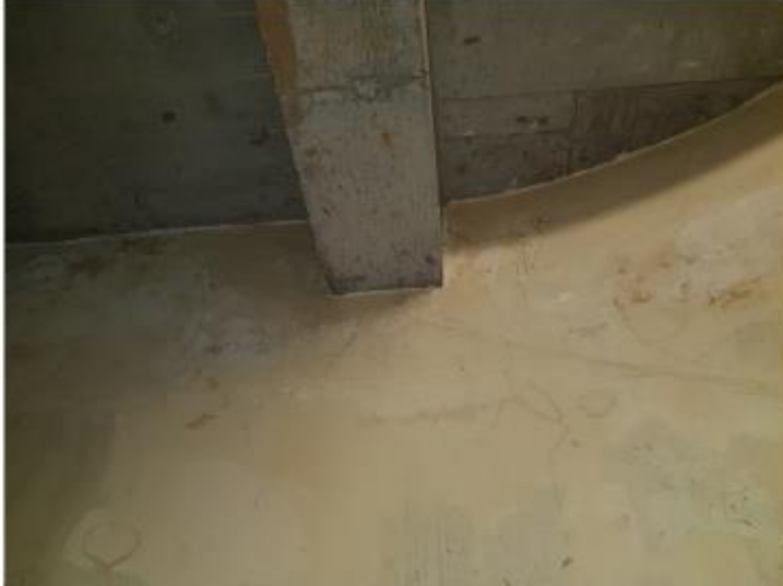
Figure 31: Damp Walls in Fire Escape
