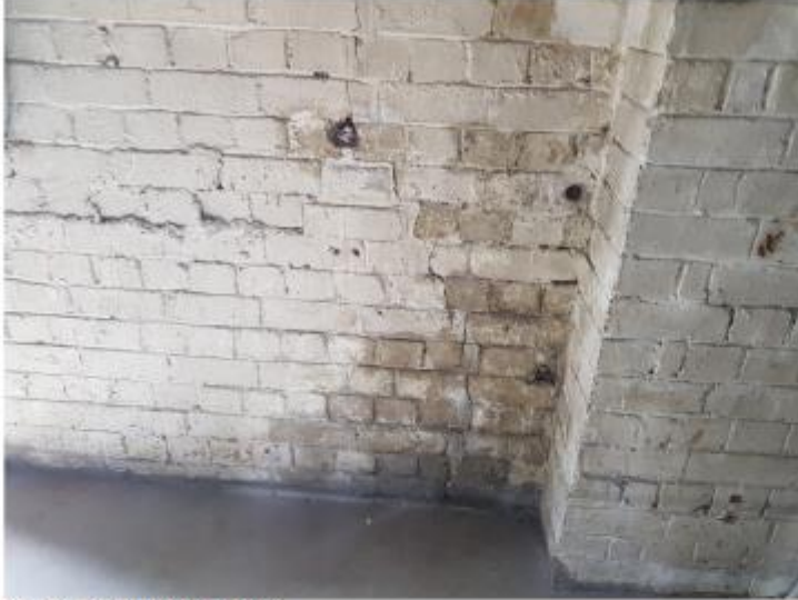
Figure 17: Cracking Around Old Embedded Fixings
