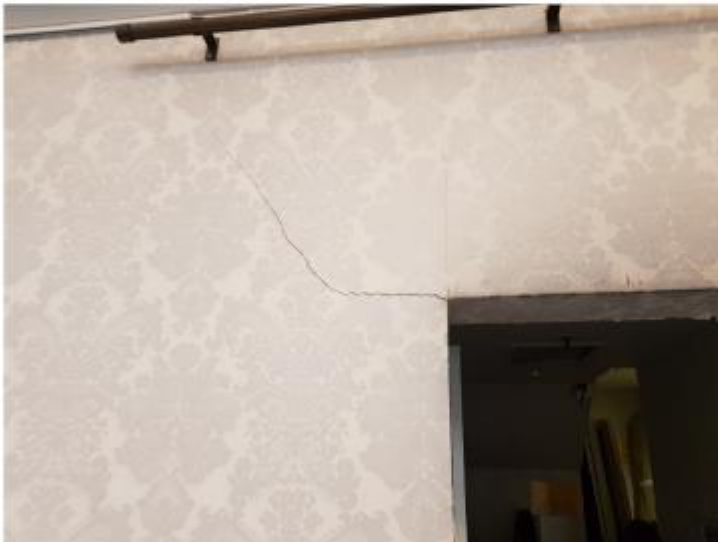
Figure 26: Diagonal Cracking in Tea Room Lintel
