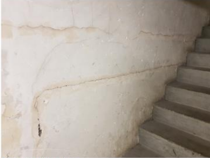
Figure 19: Cracking in Northern Fire Escape Walls
