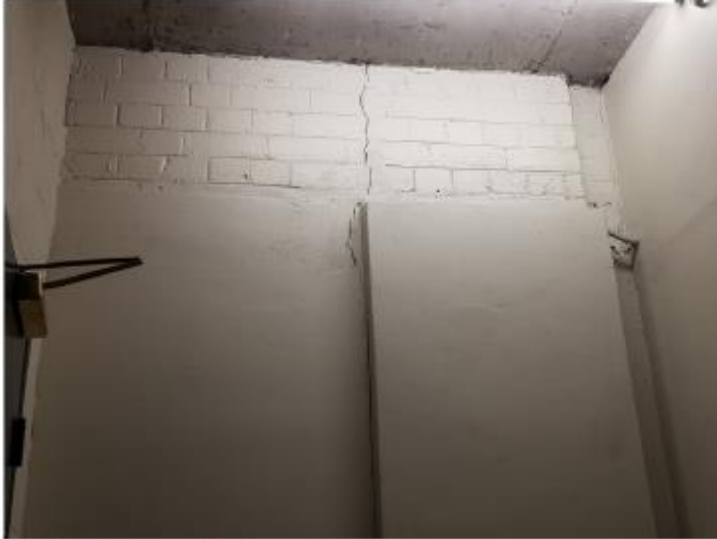
Figure 21: Vertical Cracking in Masonry
