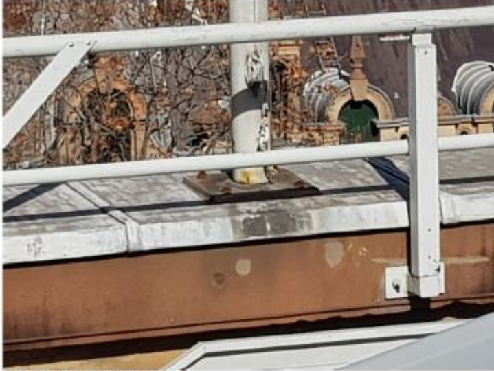
Figure 5: Corroded Flag Pole Connections South End
