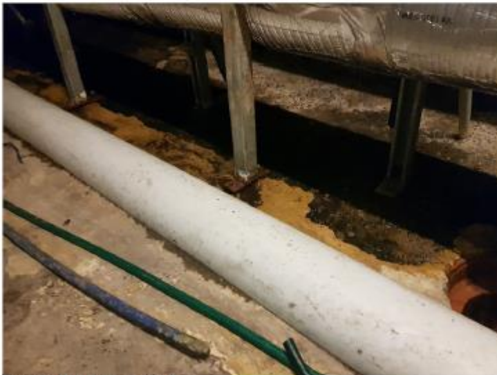
Figure 44: Ponding Water in Lower Ground Service Corridor
