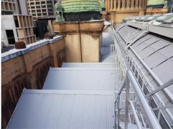
Figure 11: Typical New Access Walkways
