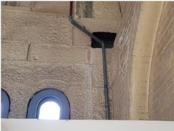
Figure 36: Water Staining From Dome Roof
