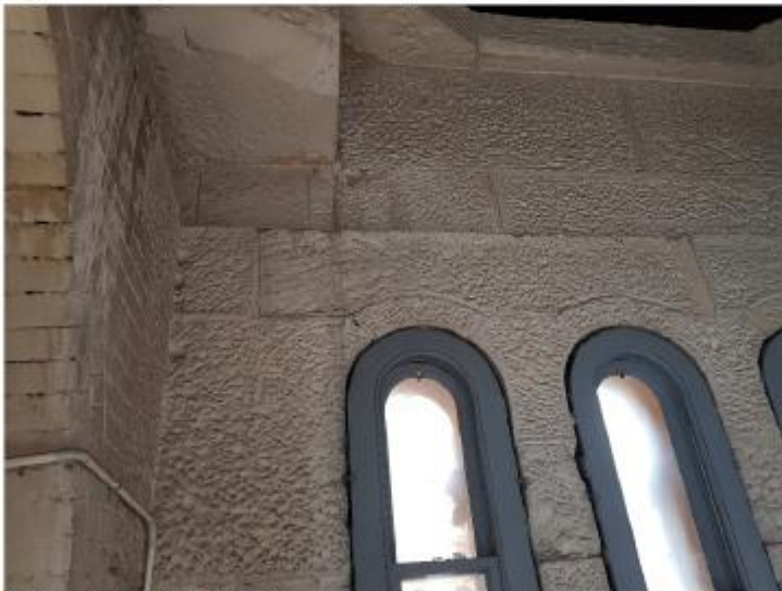
Figure 14: Diagonal Cracking Through Bed Joints Above Windows
