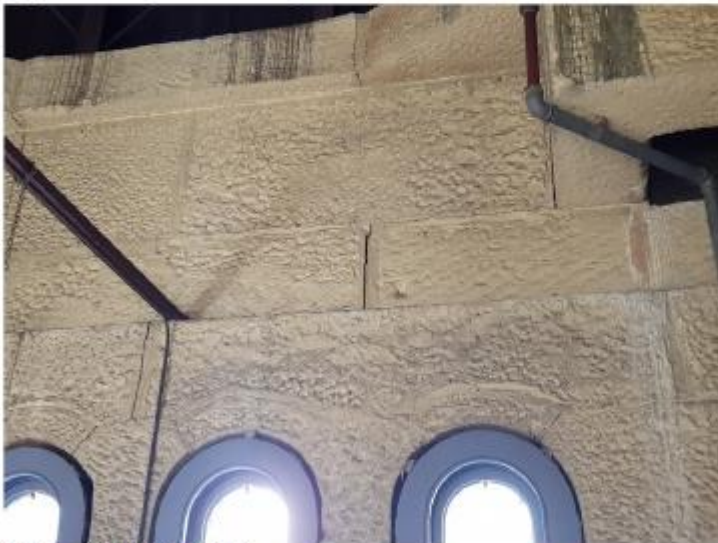
Figure 16: Diagonal Cracking Through Bed Joints Above Windows
