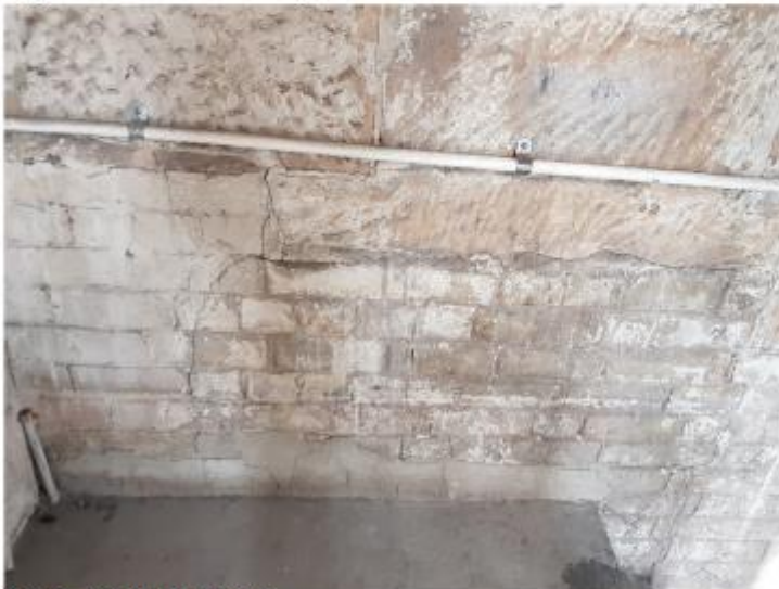
Figure 18: Vertical Cracking at Sandstone Brick Interface
