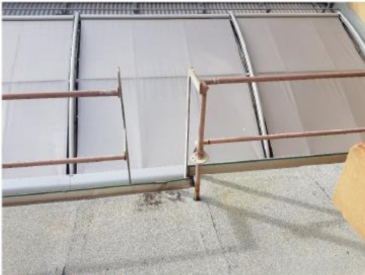
Figure 6: Balustrade North West
