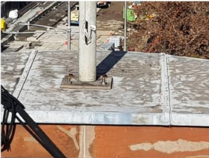
Figure 4: Corroded Flag Pole Connections South End
