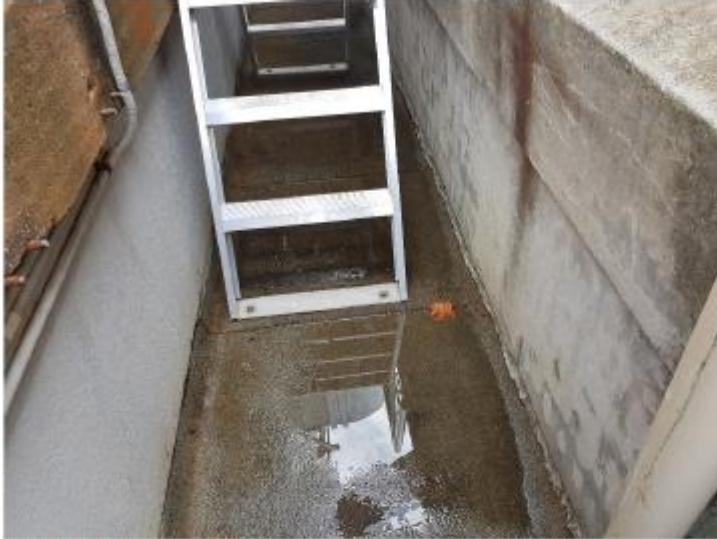
Figure 33: Ponding Water on North East Flat Roof
