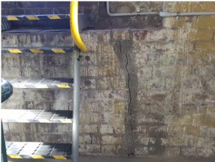
Figure 22: Vertical Cracking in Masonry
