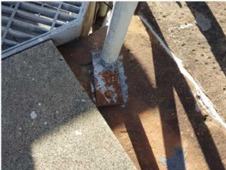
Figure 10: Corroded Connection of Access Structure South End
