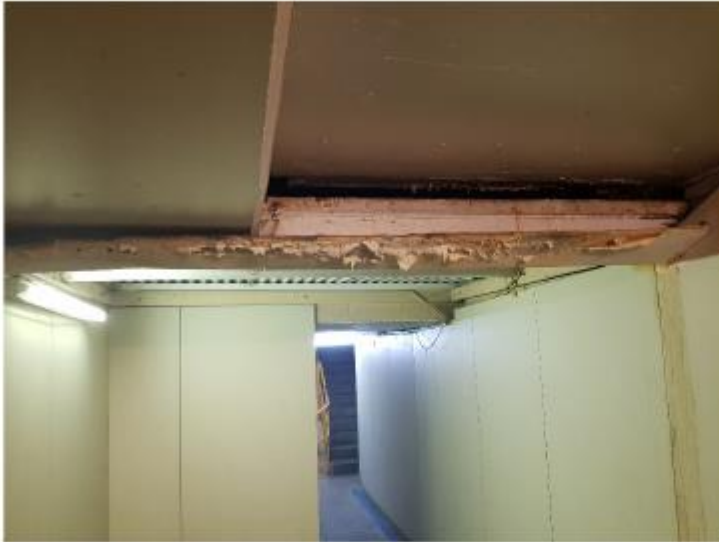
Figure 43: Water Staining Around Lower Ground Gutter in Service Corridor
