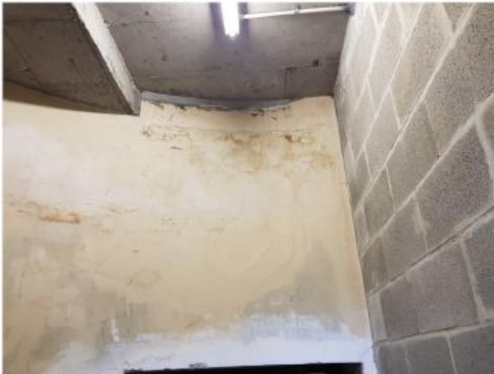
Figure 32: Damp Fire Escape Walls Under North West Flat Roof
