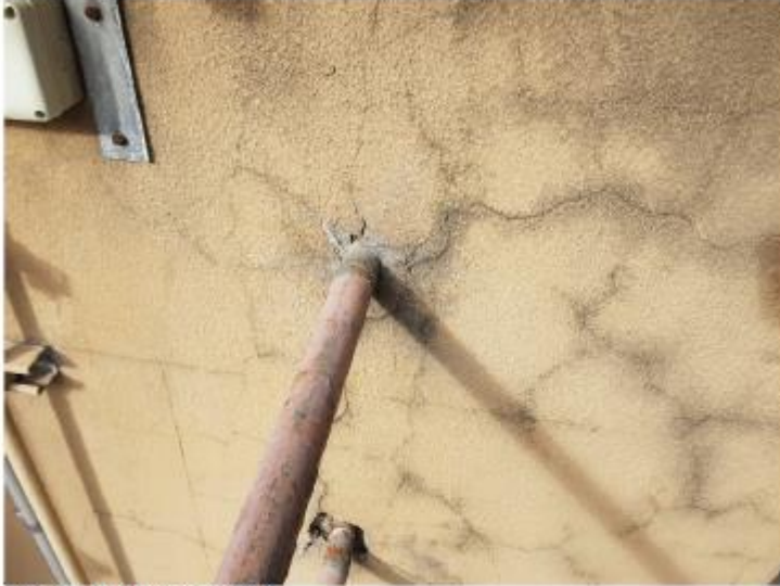
Figure 9: Cracking Around Embedded Railing
