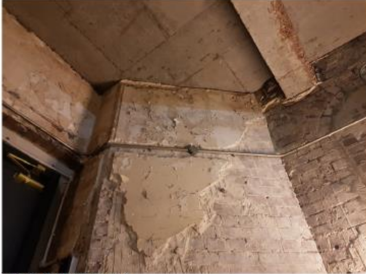
Figure 41: South Fire Escape Damp and Spalling Concrete
