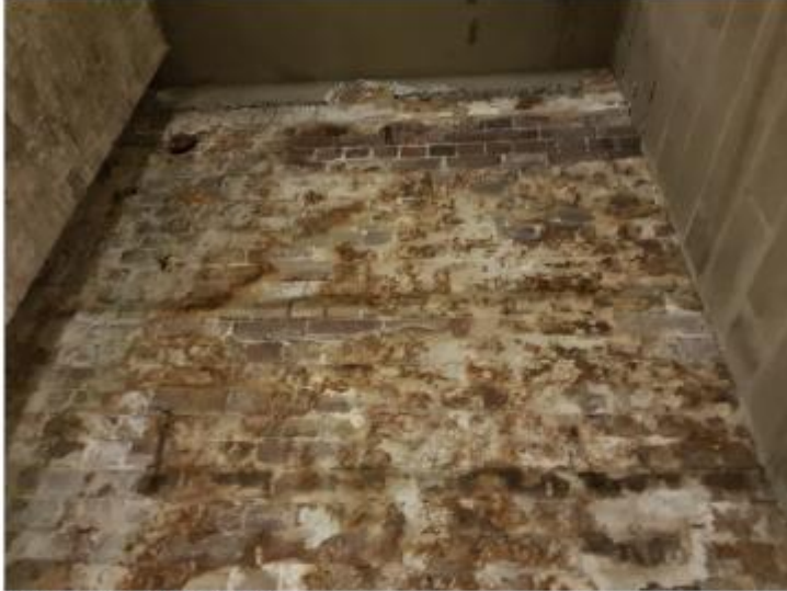
Figure 45: Damp Wall in Lower Ground Fire Escape
