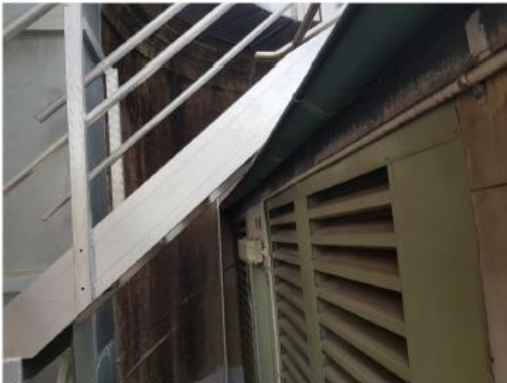
Figure 50: Bowing Gutter Above North West Flat Roof
