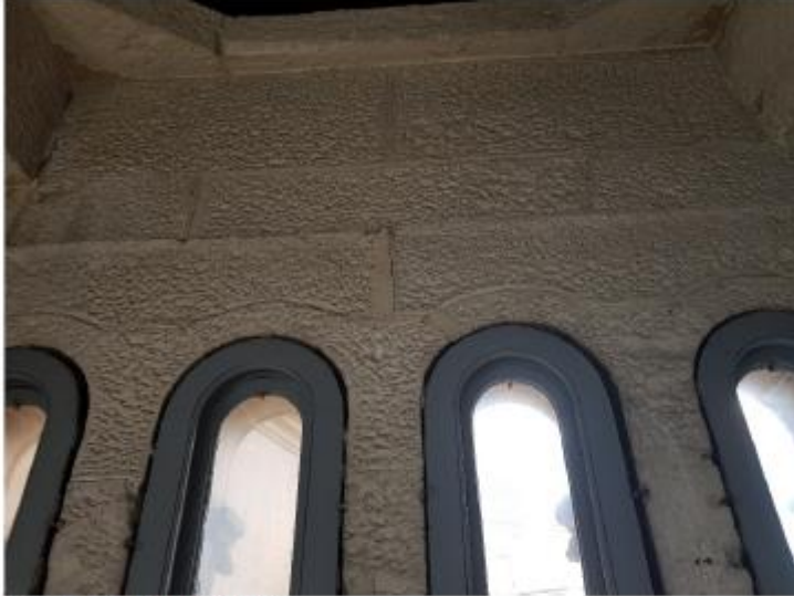
Figure 13: Diagonal Cracking Through Bed Joints Above Windows
