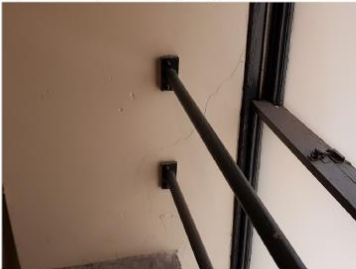
Figure 20: Cracking Around Railing Fixings
