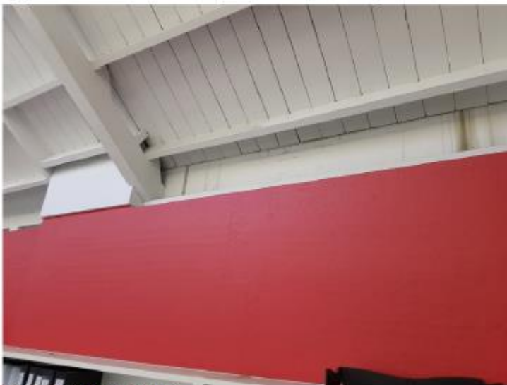
Figure 40: South East Meeting Room Water Staining
