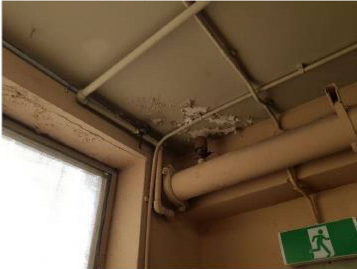
Figure 25: Cracking in Lintel
