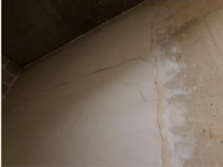
Figure 27: Fire Escape Cracking
