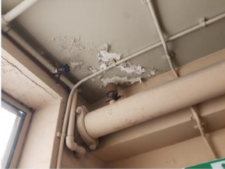
Figure 29: Spalling Concrete
