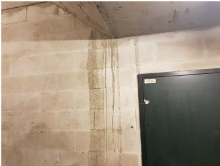
Figure 46: Signs of Water Ingress in Lower Ground Fire Escape
