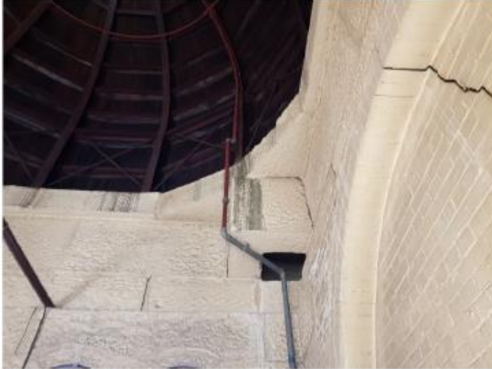
Figure 35: Water Staining From Dome Roof
