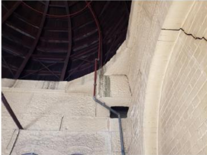
Figure 23: Vertical Cracking in Dome Masonry
