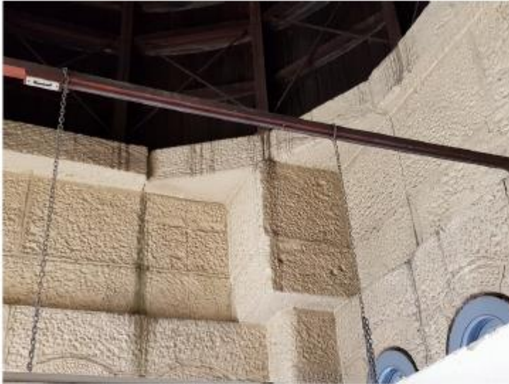
Figure 37: Water Staining From Dome Roof
