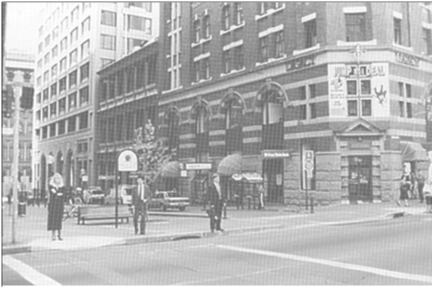
Kerb ramps at pedestrian crossing.
