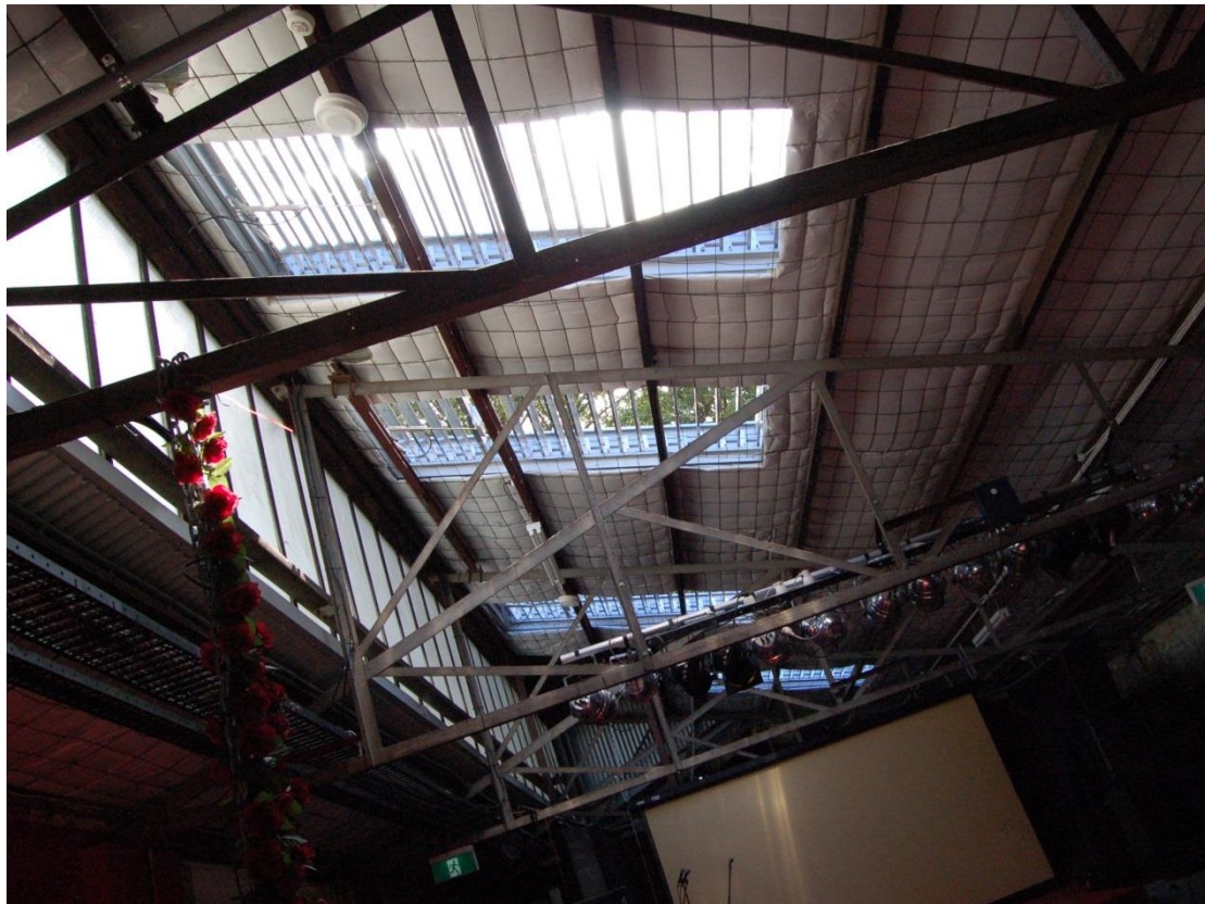
The venue's ceiling, demonstrating noise insulation and smoke extractor vents Photo: Penelope Benton
