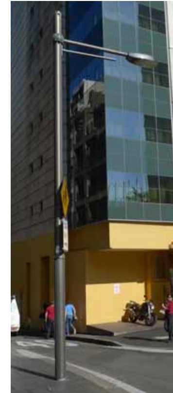
Example of ‘village’ smart pole at Darlinghurst Road, which is smaller in scale and darker in colour than the smart poles used for public lighting in the city centre.
