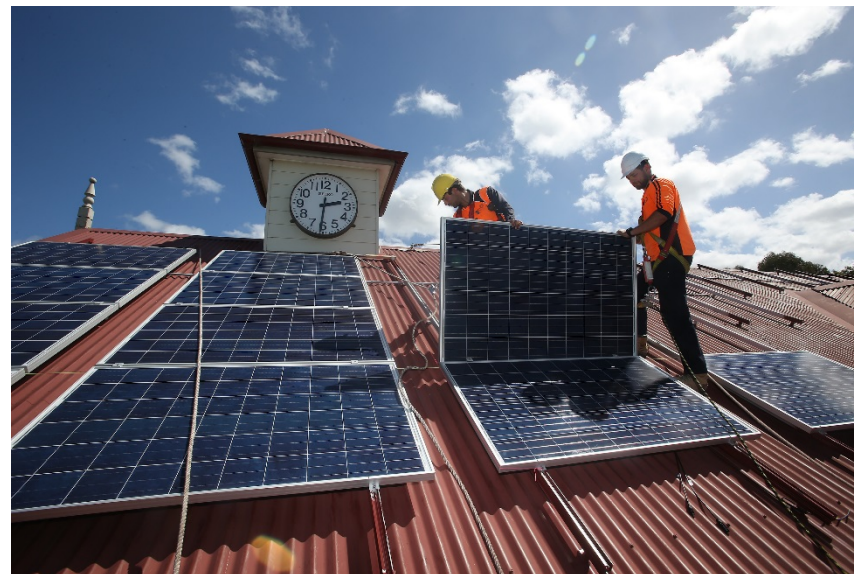
Image: Solar panels are installed on the roof of the pavilion at Sydney Park
