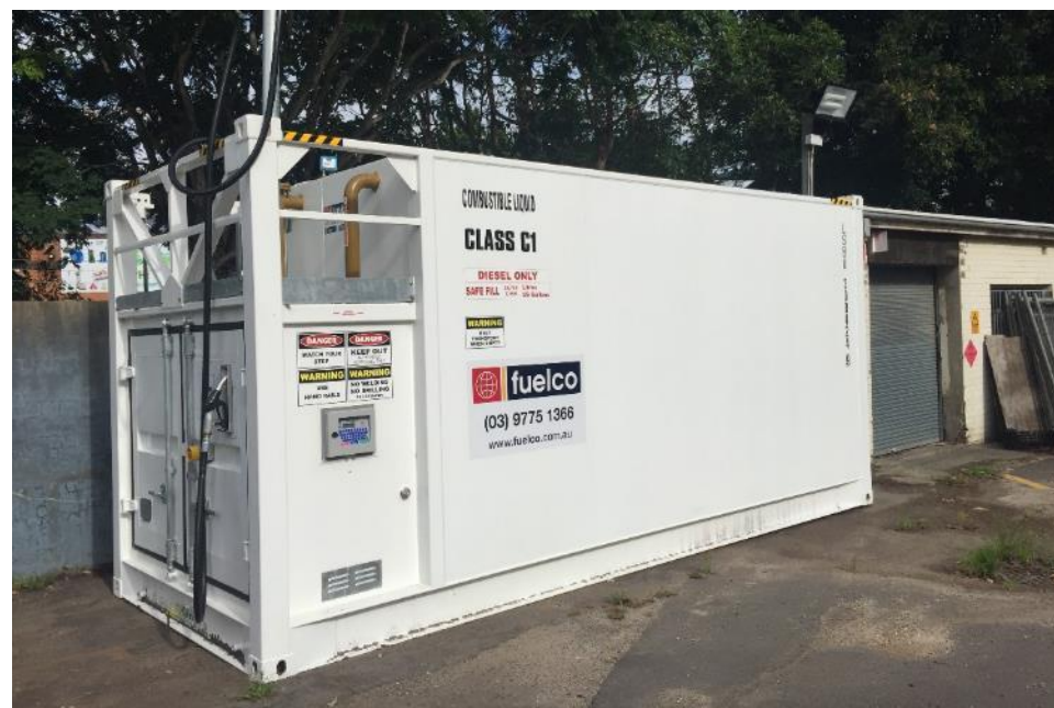
Image: New installation of bulk fuel tank at Parks Nursery St. Peters
