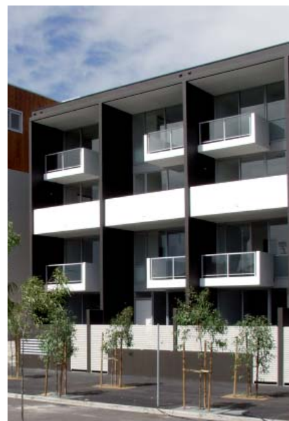
Figure 24: Maisonette type dwellings Victoria Park (Turner Associates)
