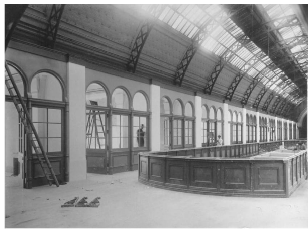
Figure 50 –Balustrades of the upper levels were enclosed with timber cladding, 1918
