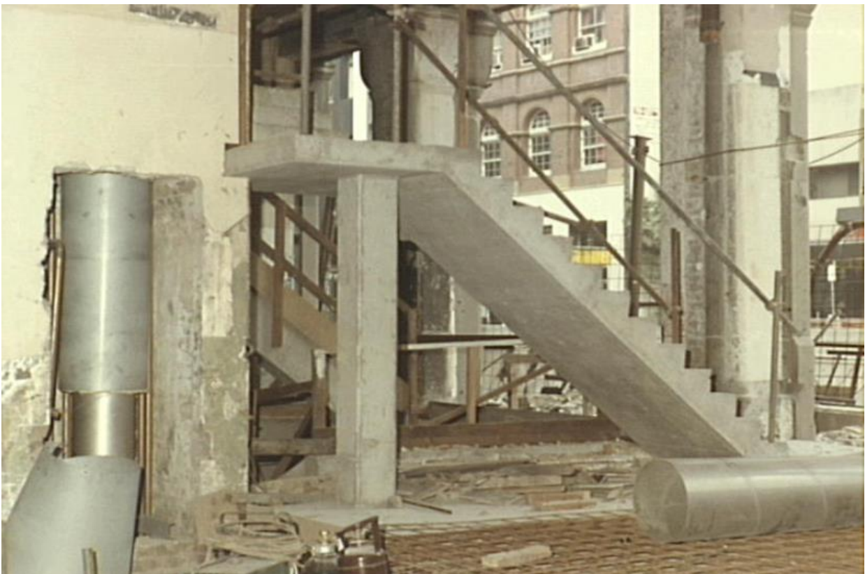
Figure 78 – Concrete stairs leading out to York Street
