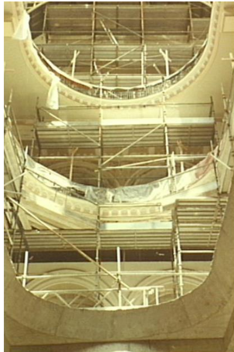
Figure 75 - Looking up through the newly recovered central dome area prior to the installation of
