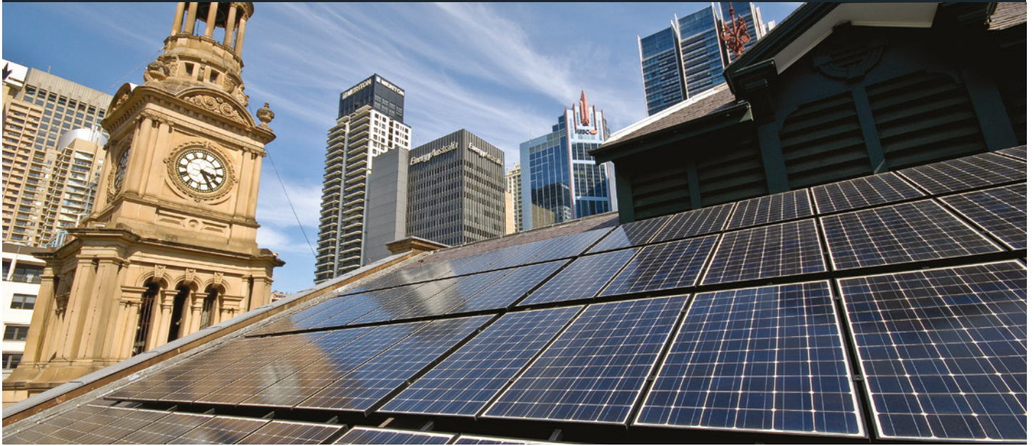
Town Hall House solar panels, October 2010. Photographer: Paul Patterson
